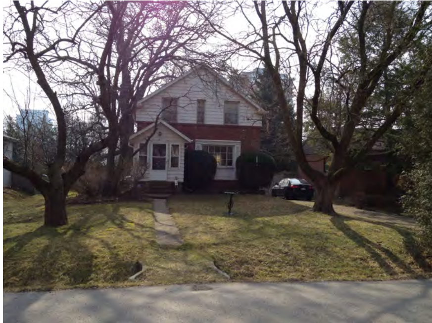
Neighbouring dwelling across Oriole Ave from subject site
