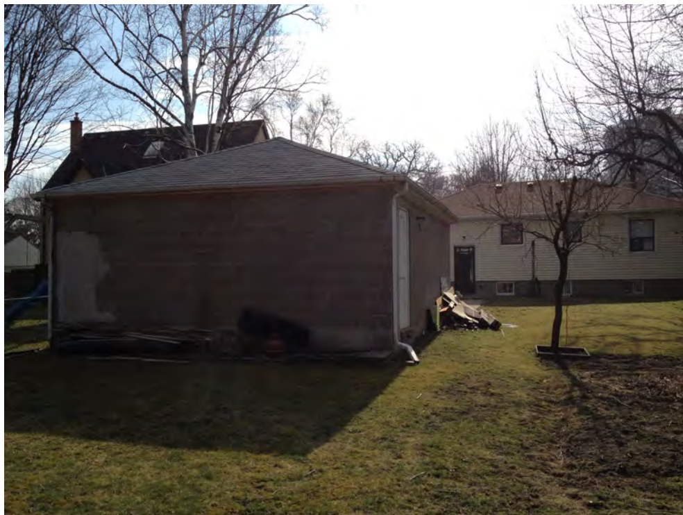
Rear elevation (north), showing garage rear
