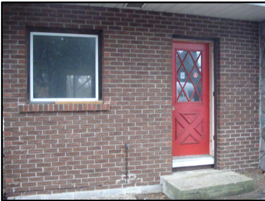
Side door entry to Kitchen
