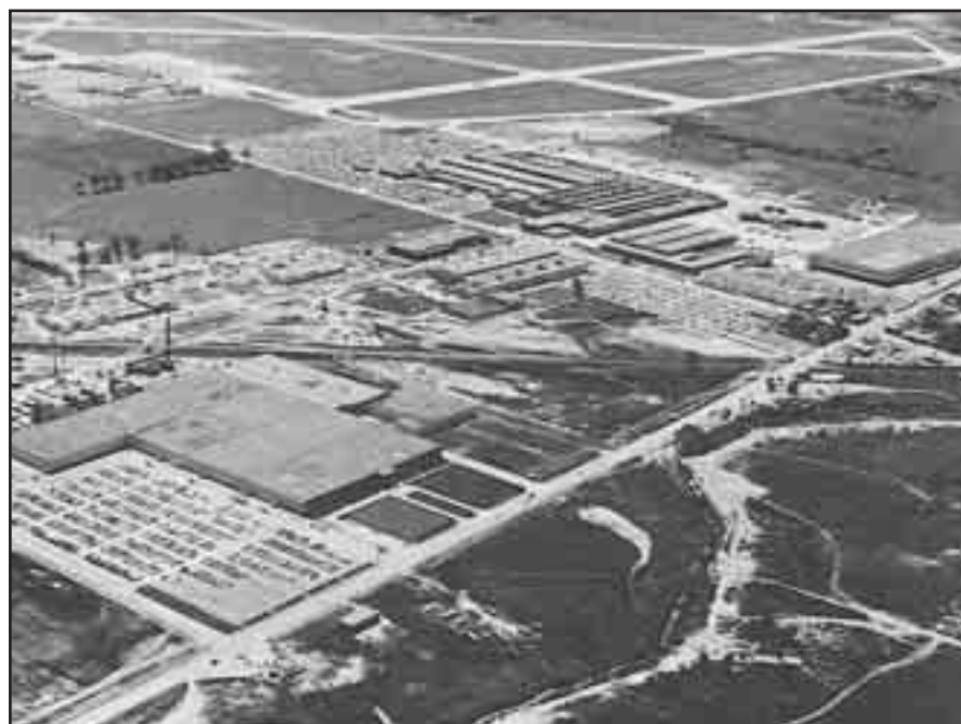
▲ The A. V. Roe Canada Complex, mid 1950s: Orenda Jet Engine Plant, upper right, Avro Aircraft Plant, top left, the Toronto Airport Terminal Building (Magellan Aerospace Corporation)
