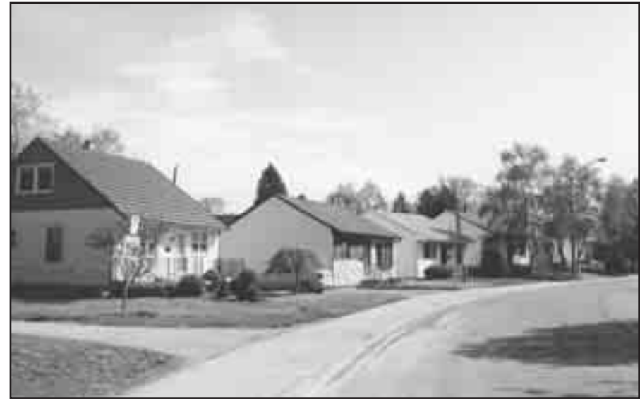
▲ Victory Village Houses, 2006
