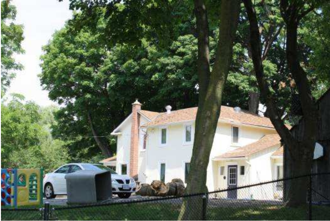
1100 Old Derry Road West, west elevation.
