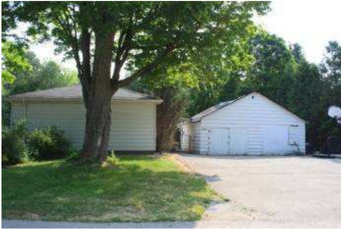
7067 Old Mill Lane, the west façade and outbuilding.
