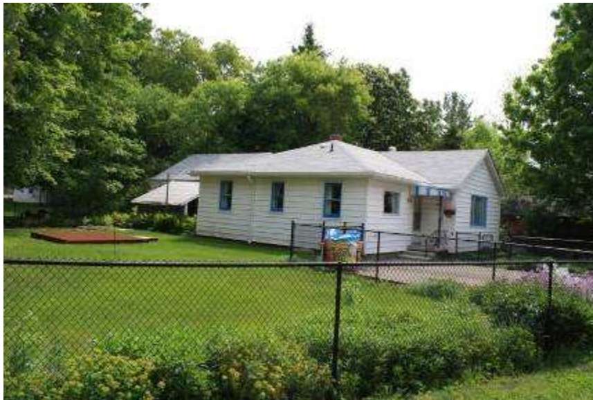
7035 Old Mill Lane, north and west facades.
