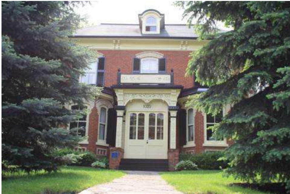
Graham-Pearson House, front, north elevation.
