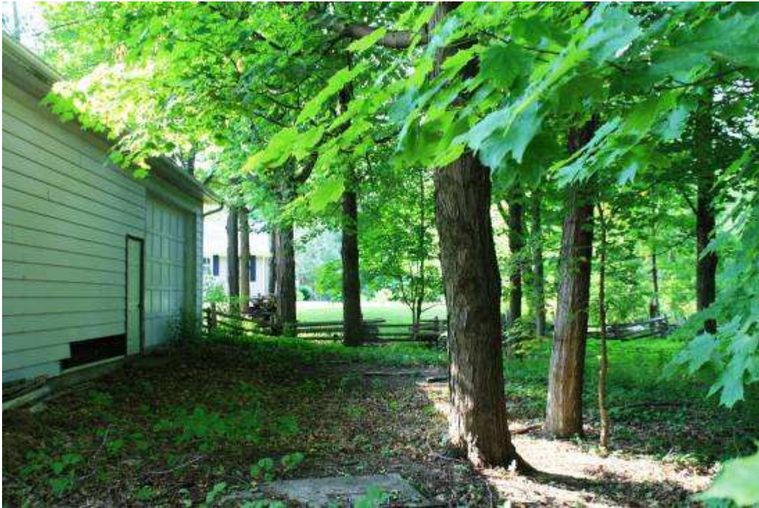
7060 Pond Street rear façade.
