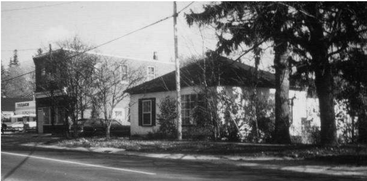
Lambe residence in 1974 prior to the renovations and addition.
