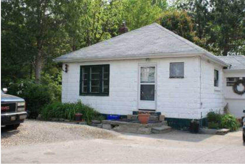
Concrete block residence at 1056 Old Derry Road
