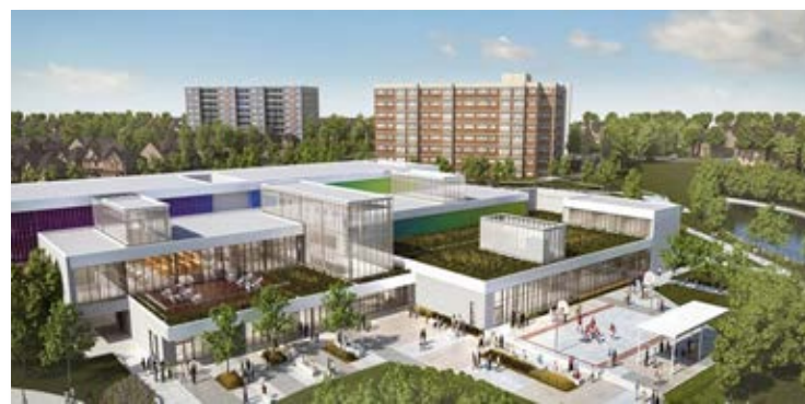
2018 Mississauga Urban Design Award of Excellence and the 2018 Mississauga Urban Design Award of 'Healthy by Design': Meadowvale Community Centre and Library
