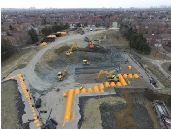
Installation of storage chambers at Eastgate Park
