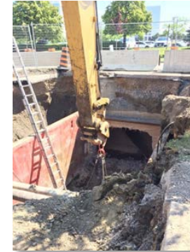
Installation of storm pipe infrastructure
