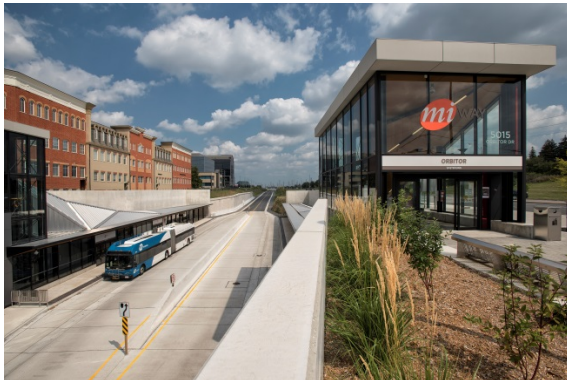
The completed Transitway at Orbitor Station
