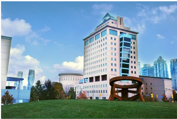
ENERGY STAR certification for City Hall
