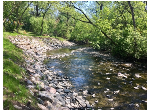
Watercourse bank stabilization at failed storm outfall
