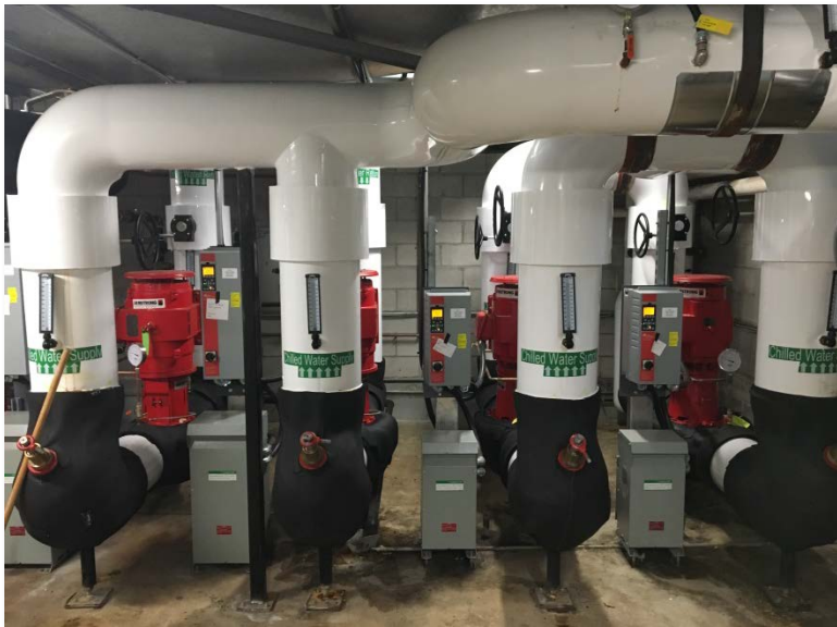
Mississauga City Hall - Cooling Tower Replacement & Chilled Water Plant Upgrades
