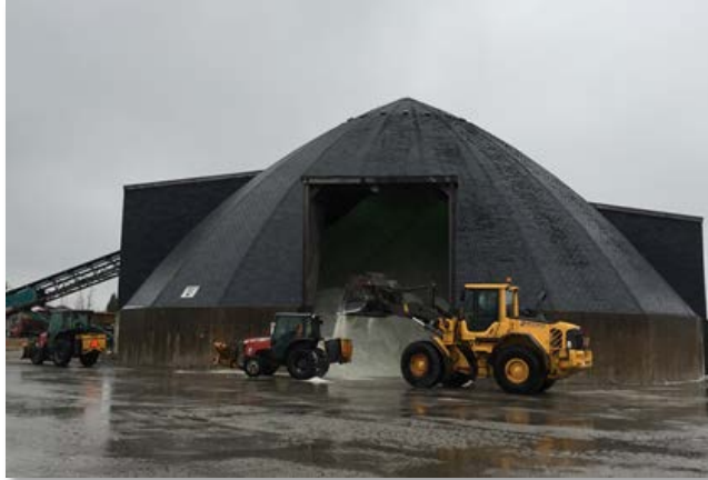
Salt storage dome at the Mavis Works Yard
