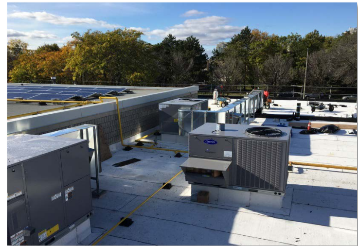
Burnhamthorpe Community Centre - HVAC and Roof Upgrades
