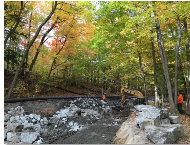
Erosion control projects improve the condition of the City's watercourses
