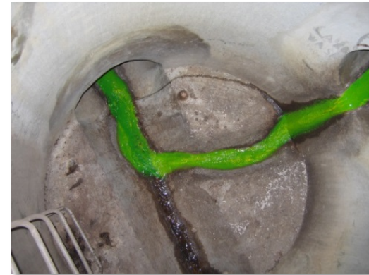
Storm Sewer dye test to confirm sanitary cross connections
