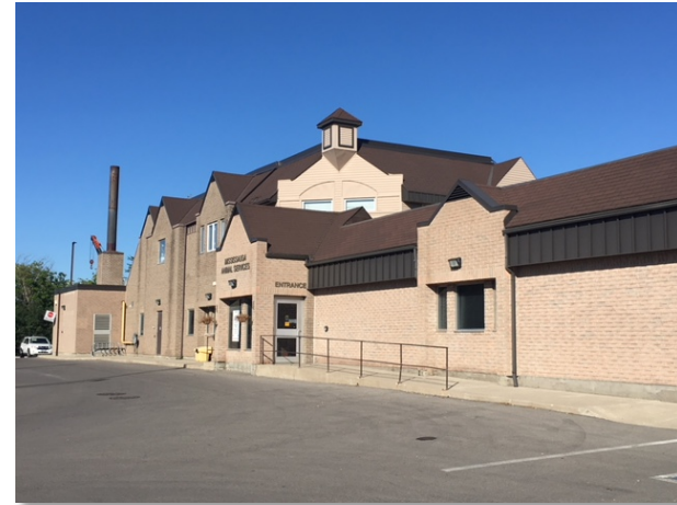
Feasibility Study underway to optimize current Animal Services Centre Facility
