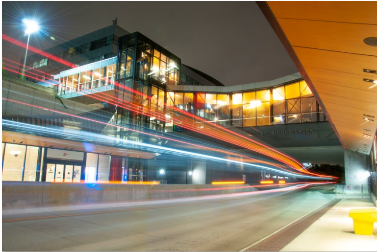
Mississauga Transitway – Etobicoke Creek Station
