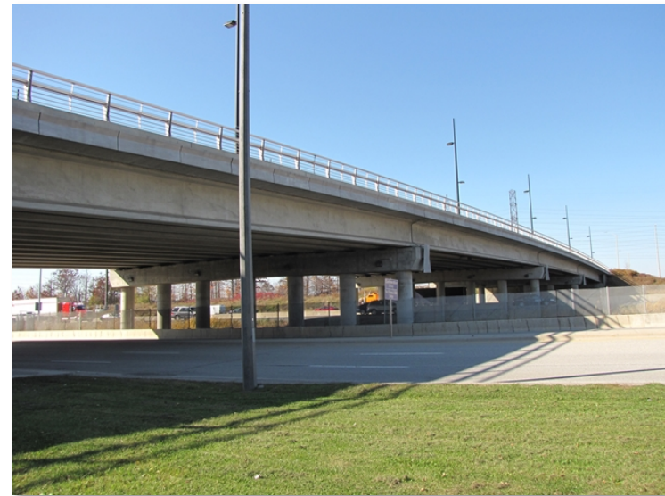
Confederation Parkway bridge over Centre View Drive
