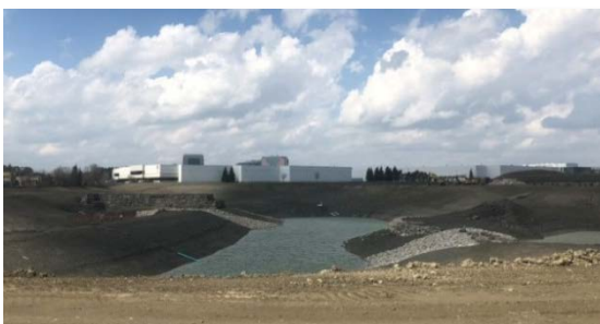
Matheson Boulevard Stormwater Pond
