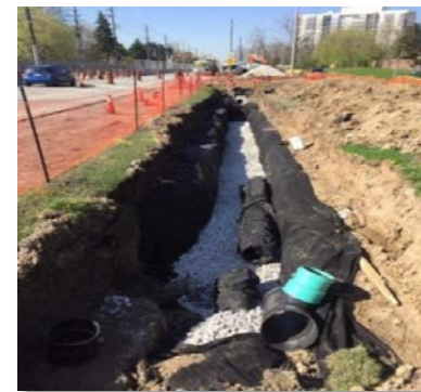
Burnhamthorpe Road East Boulevard
