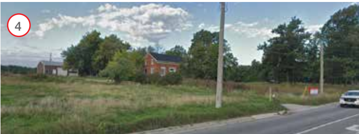
Figure 1.2e - Northwest view of the heritage house from Ninth Line
