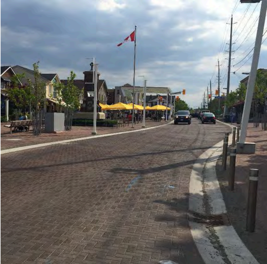
FIGURE 4.9 - A Community Improvement Plan could potentially be used to improve streetscape. In the above example from the Streetsville Neighbourhood in Mississauga, streetscape improvements were made to add special street pavers, bollards, and pedestrian street furniture.
