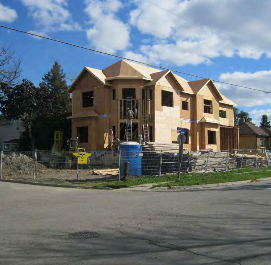
FIGURE 4.8 - An example of infill residential housing under construction in Malton.
