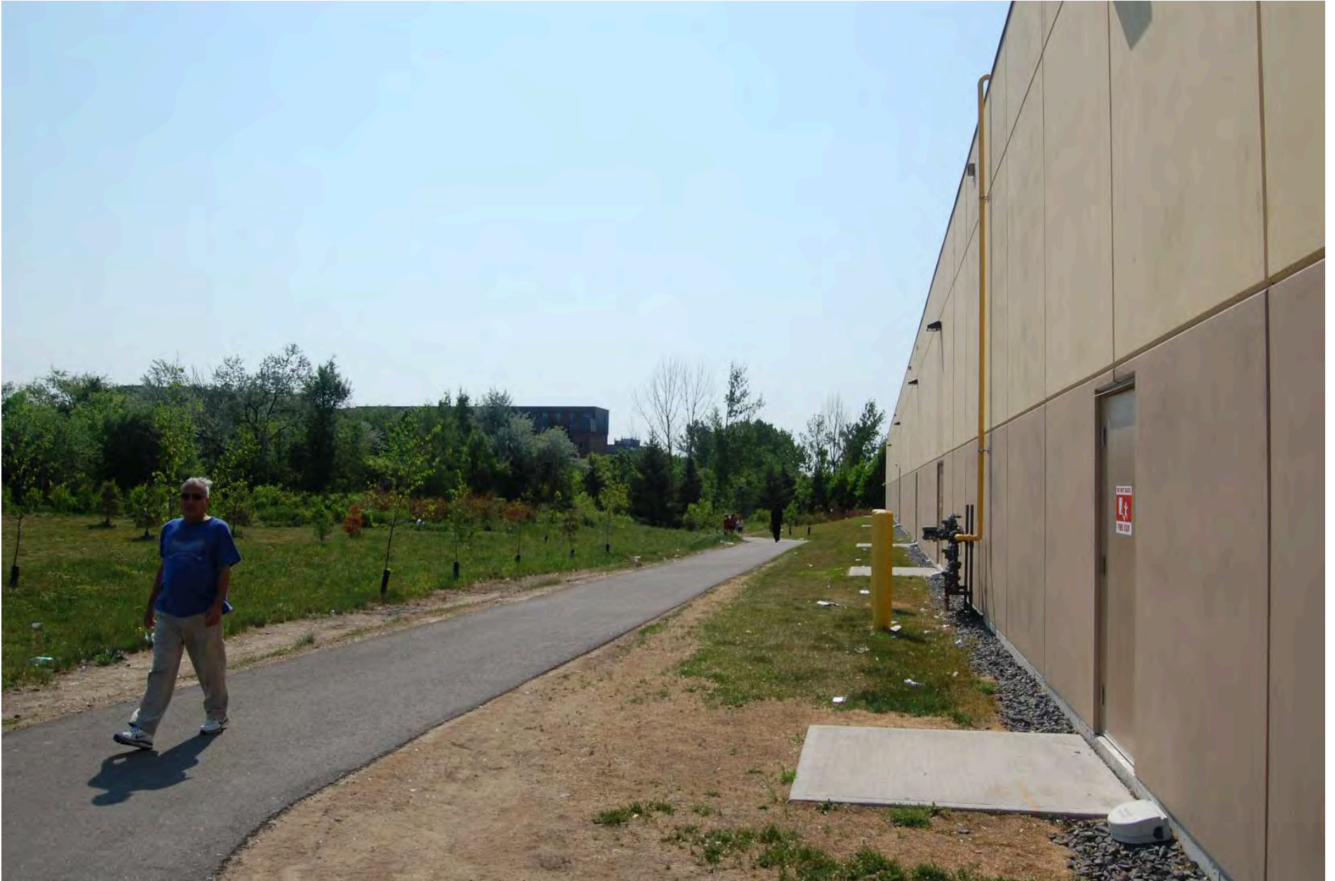
FIGURE 3.11 - Rear of Westwood Mall (Before): Many residents use this walkway to travel from the Malton Greenway to the Westwood Transit Terminal, or as a connection to Walmart.
