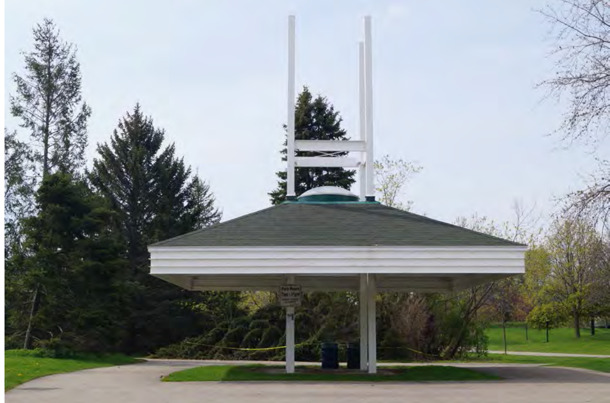
6.1 North elevation, shade structure, 2018/05/14
