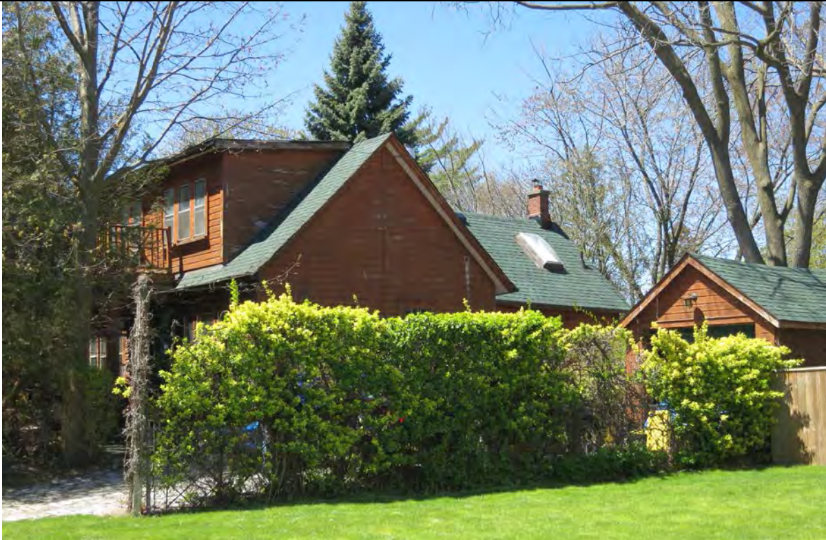
6.2 Northwest corner and front yard, 2017/05/08
