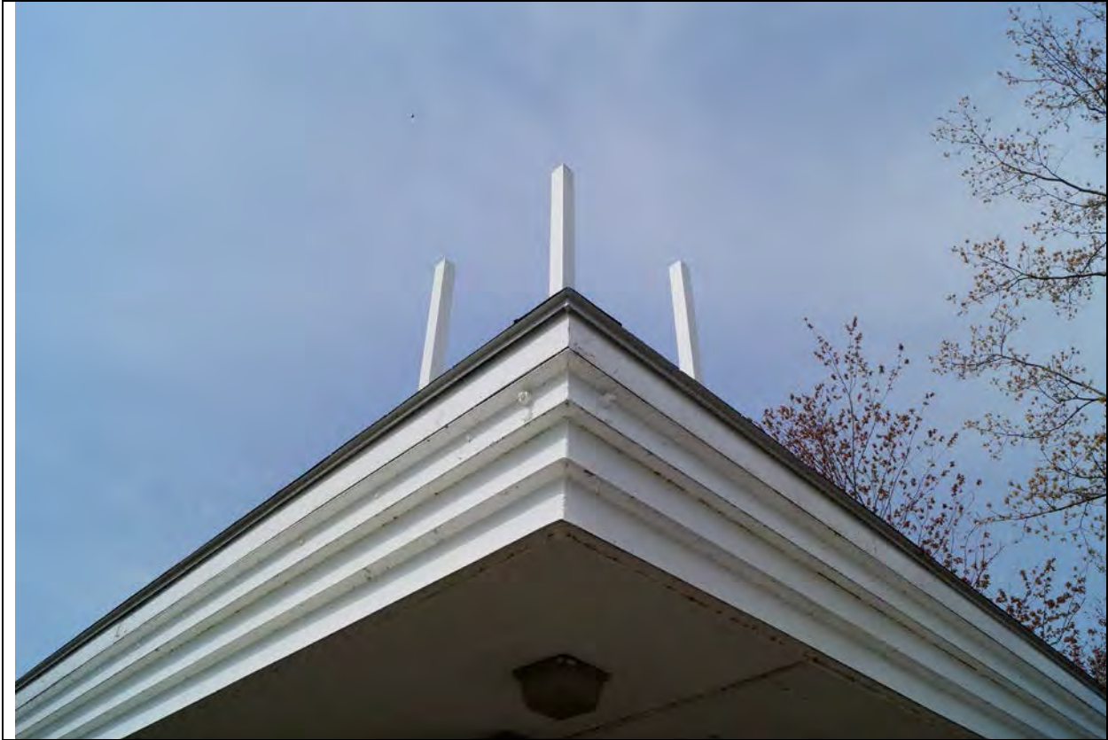
6.5 Detail, public washrooms, 2018/05/14
