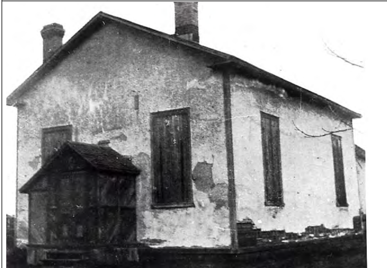
6.4 Northwest corner of the Wesleyan Methodist Church, early twentieth century.
