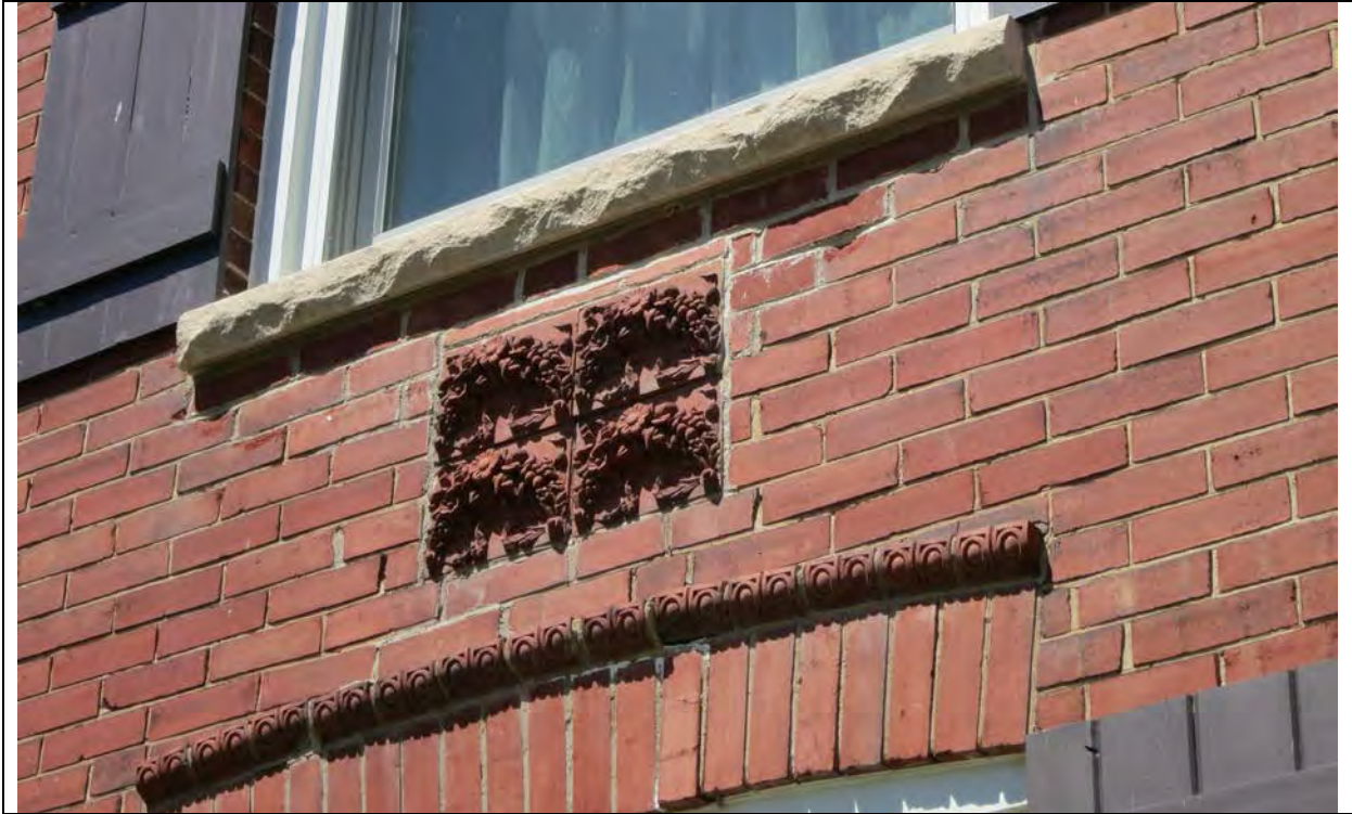
6.4 South elevation decorative terracotta brick profiles, 2017/05/08
