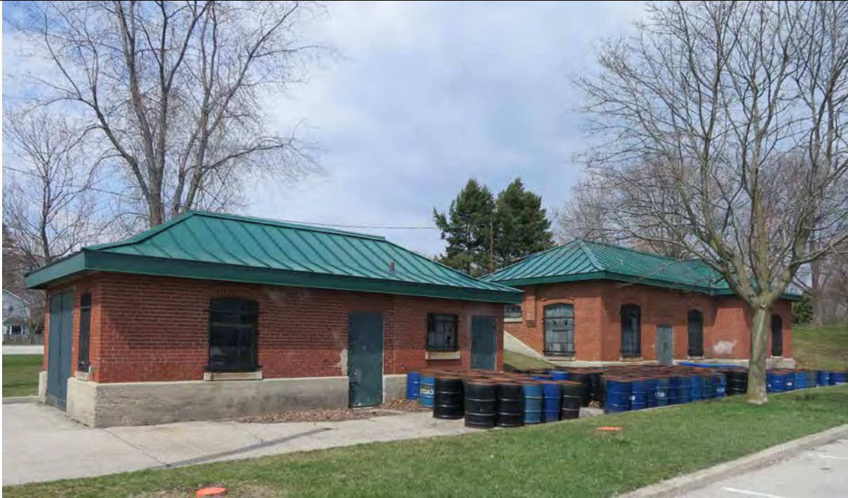
6.1 South elevation, pumping station, 2017/05/08
