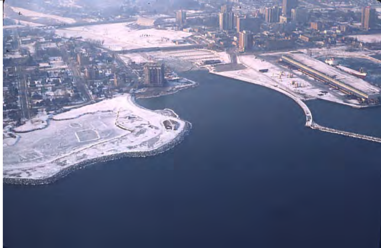
6.2 Aerial view of 35 Front Street South under construction, 1972
