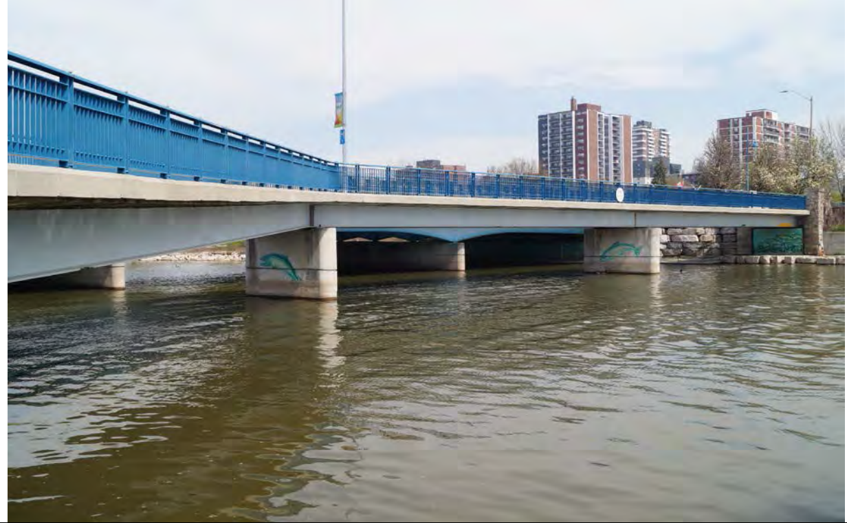
6.1 South elevation, pedestrian bridge, 2018/05/14
