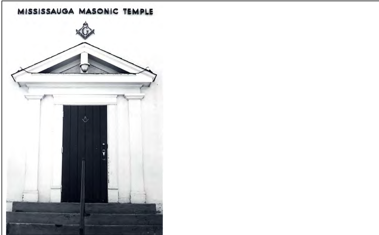
6.3 Entrance door detail, 1976
