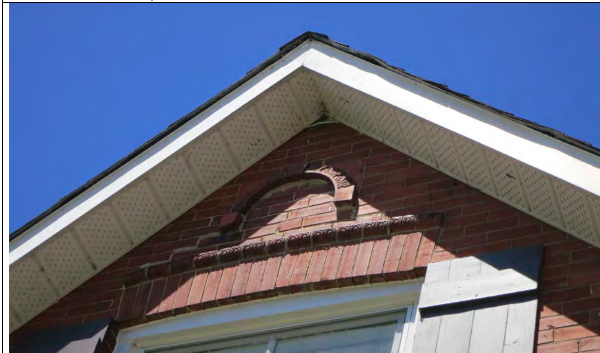
6.3 South elevation decorative terracotta brick profiles, 2017/05/08
