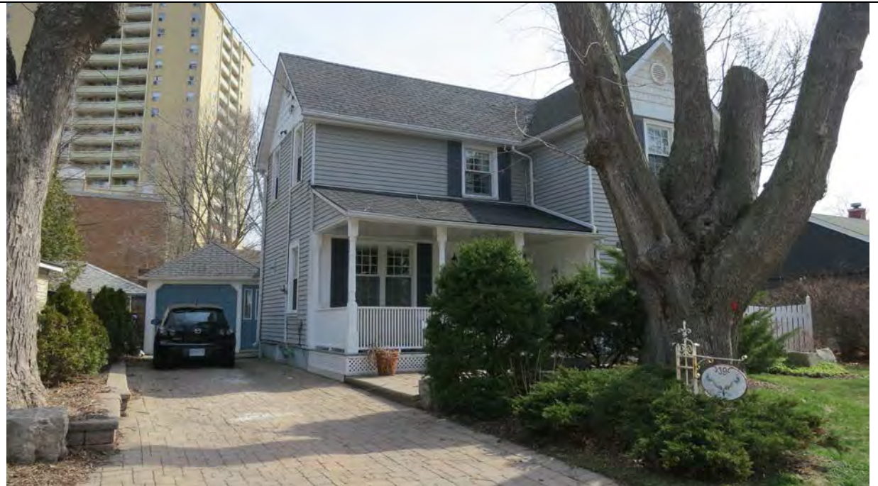
6.2 Northwest elevation, detached garage, 2017/04/10
