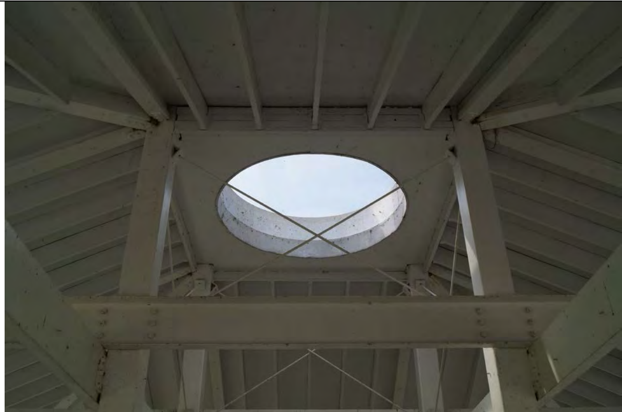
6.2 Detail, shade structure, 2018/05/14
