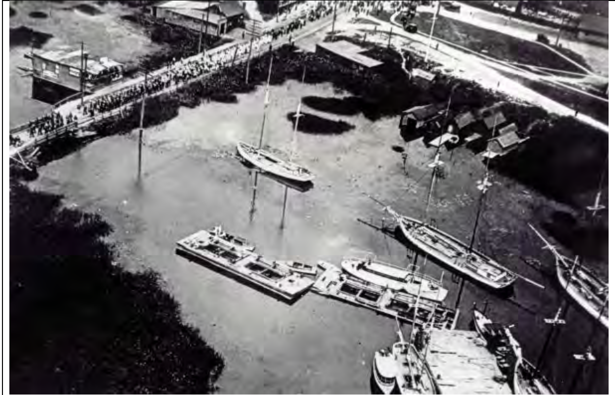
6.3 Aerial view of bridge (now replaced), 1919
