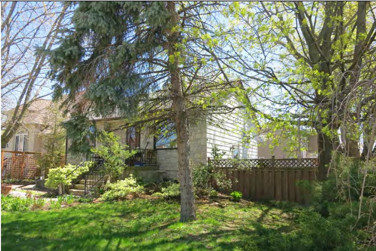
6.2 Northwest corner and front yard, 2017/05/08
