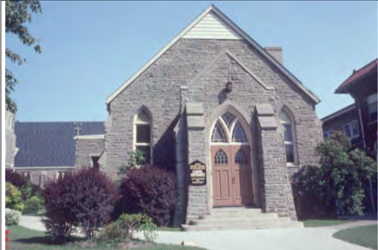
6.3 North elevation detail, 1980
