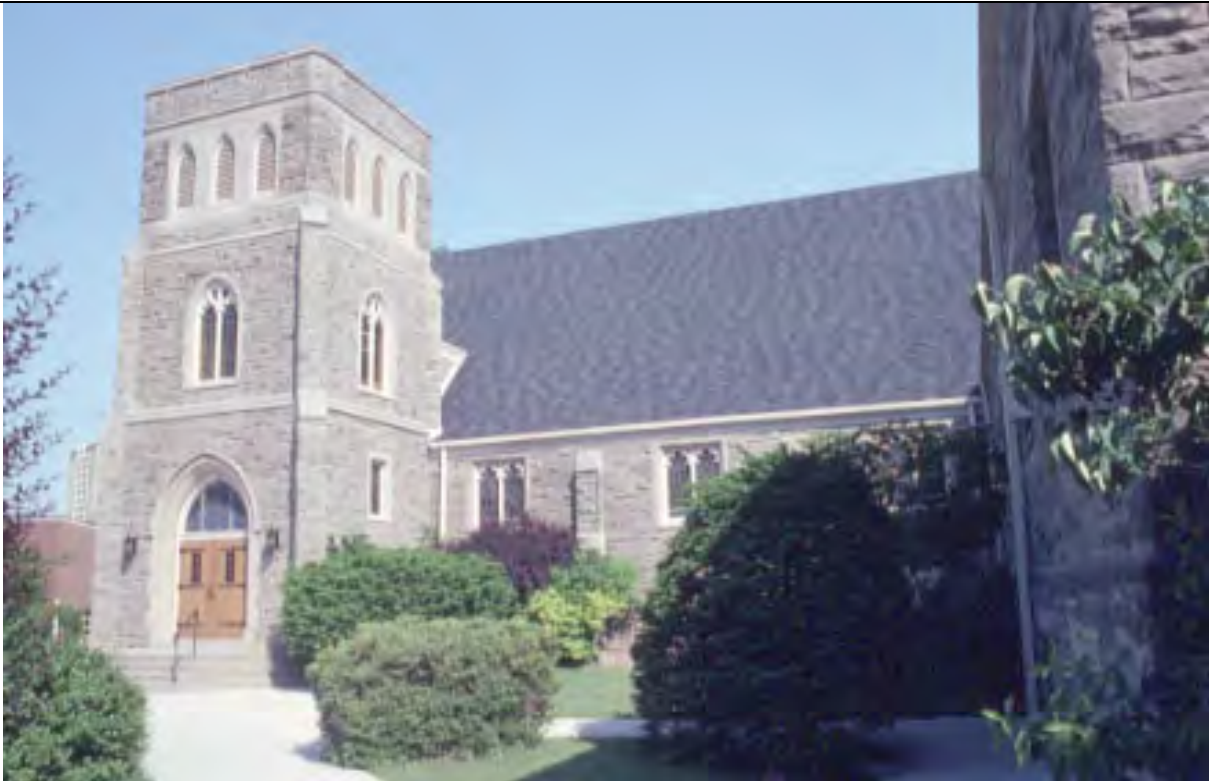
6.2 North elevation detail, 1980
