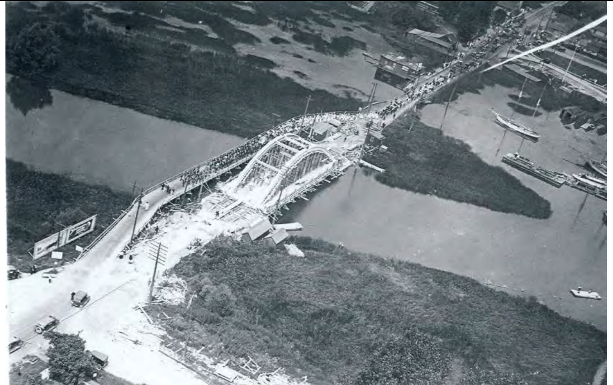
6.2 Construction of two-lane bowstring bridge (now replaced) with temporary bridge to the left, 1919.
