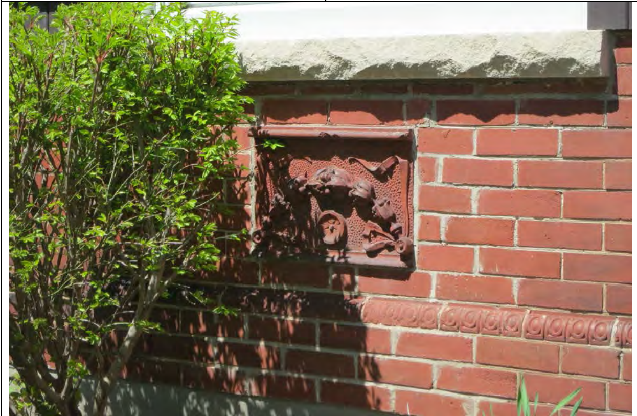
6.5 South elevation decorative terracotta brick profiles, 2017/05/08
