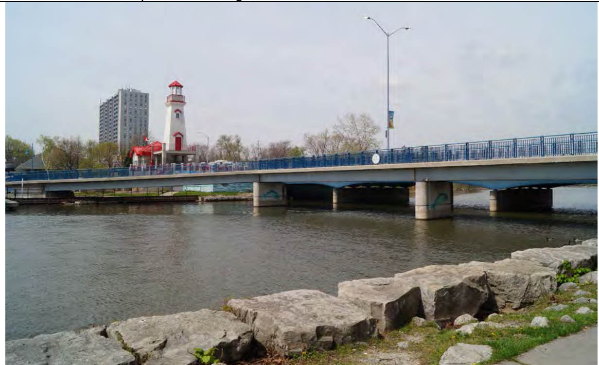
6.2 South elevation, pedestrian bridge, 2018/05/14
