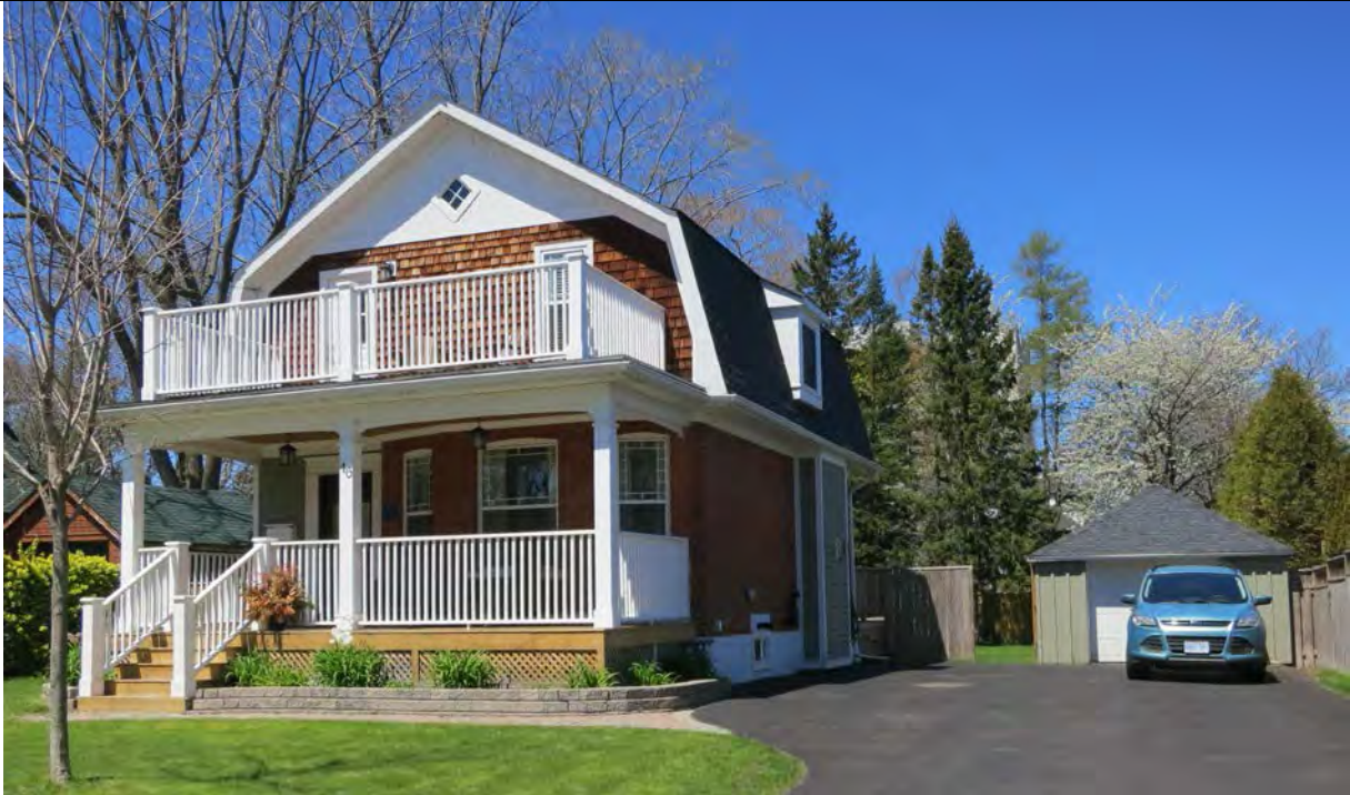
6.2 Northeast corner and detached garage, 2017/05/08
