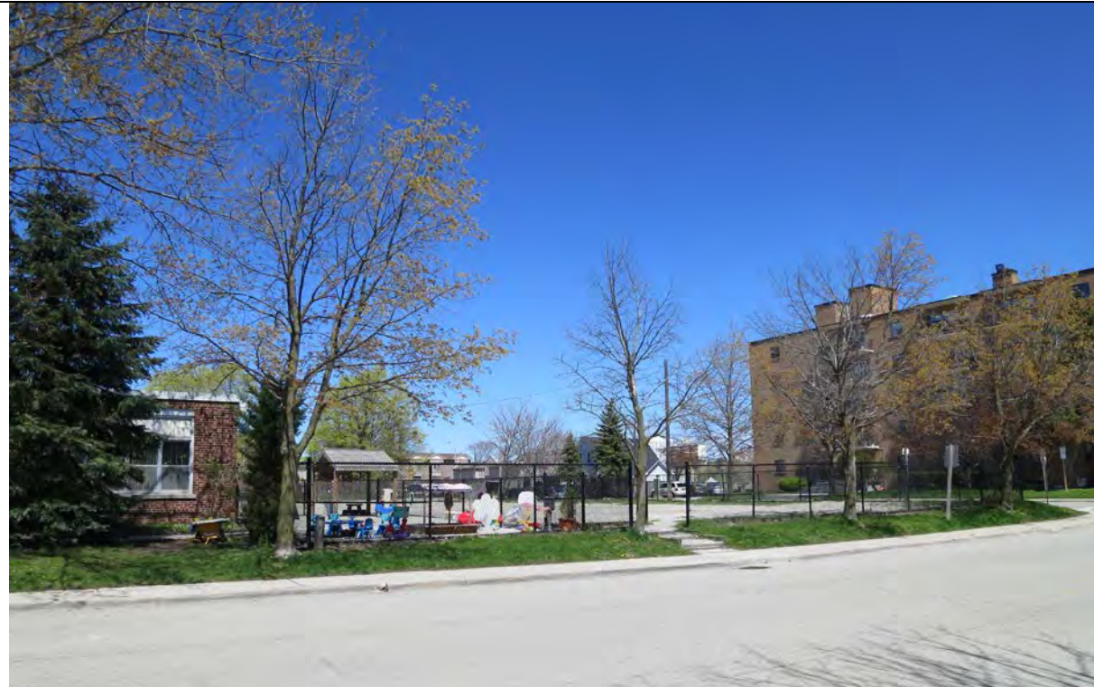
6.2 South elevation of school yard, 2017/05/08
