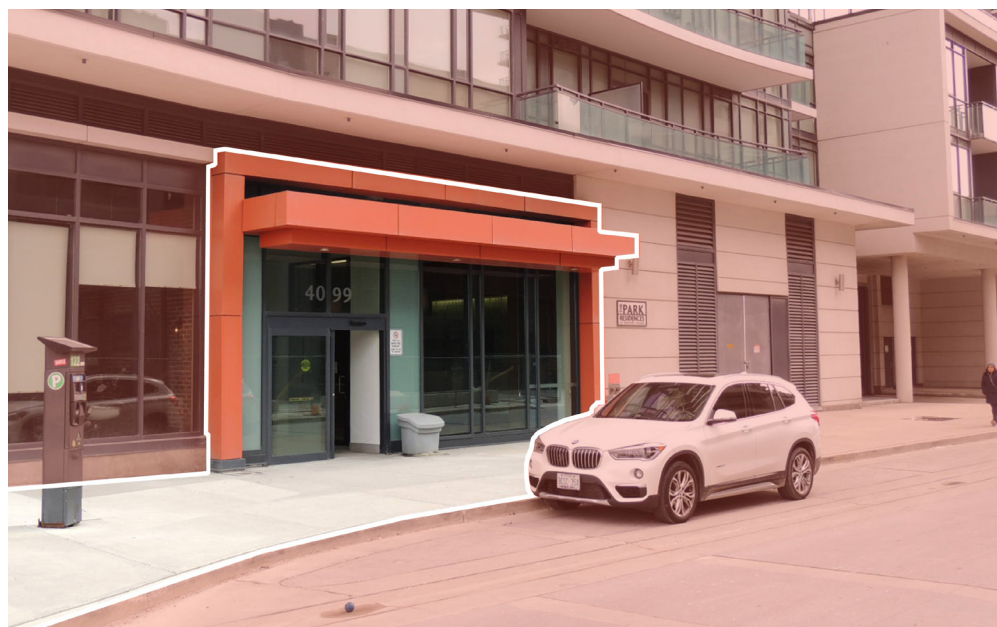
Figure 5: Prominent building entrances. Downtown Mississauga, Curran Place & Brickstone Mews
