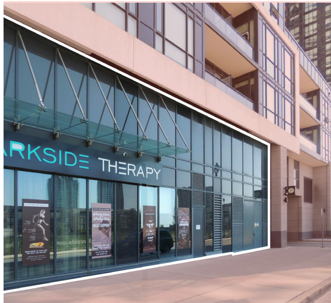
Figure 29: Transformer vault should be integrated into the design of buildings. Downtown Mississauga, Curran Place & Brickstone Mews
