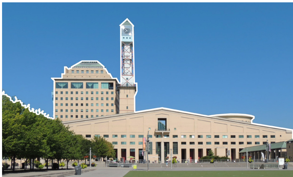
Figure 56: Tall building proposals will not compromise important view corridors or silhouettes associated with the Mississauga Civic Centre/City Hall. Mississauga Downtown, Celebration Square, Burnhamthorpe Rd W& Living Arts Centre
