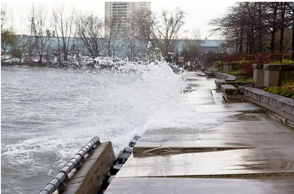
Figure 76: Heavy rains and high water hit Port Credit waterfront trail hard Mississauga, Lake Ontario Image Credit: https://www.mississauga.com/
