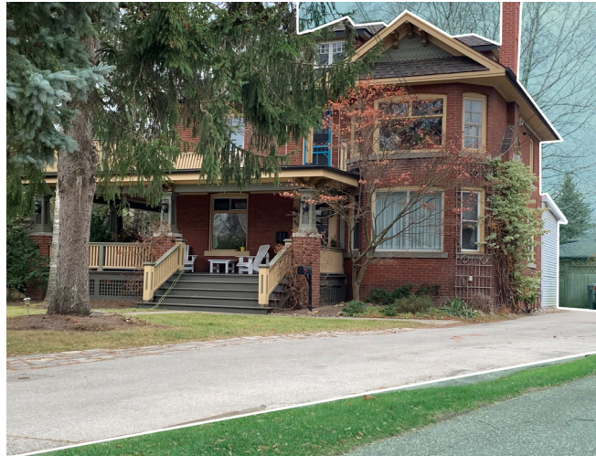
Figure 77: Example of brick material Mississauga, Wesley Ave and Park St W
