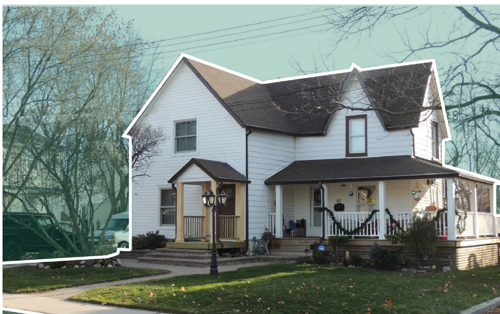
Figure 67: Example of structures in the Historic Village of Port Credit. Mississauga, John St S
