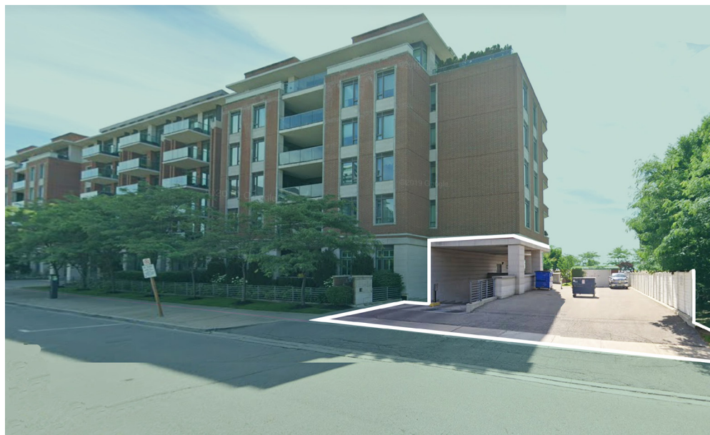
Figure 71: Loading should be located underground, internal to the building or to the rear of the buildings.
