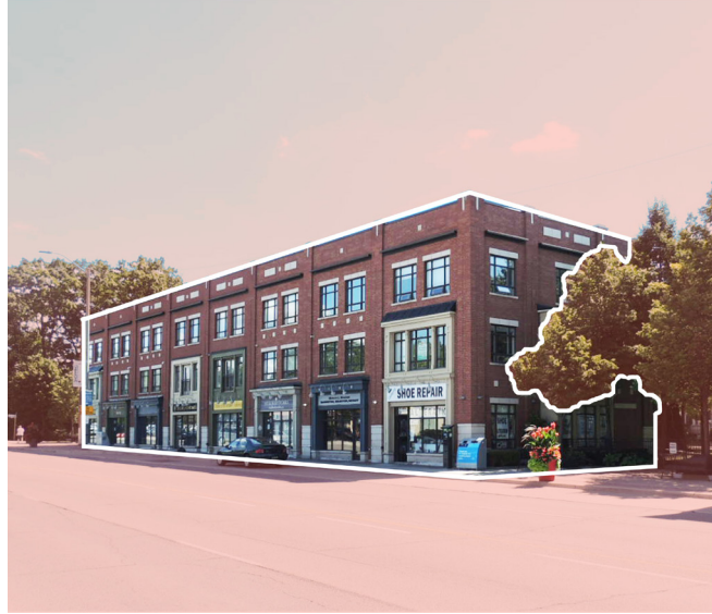
Figure 18: Image of the existing mainstreet building. Mississauga, Lakeshore Rd E and St Lawrence Dr
