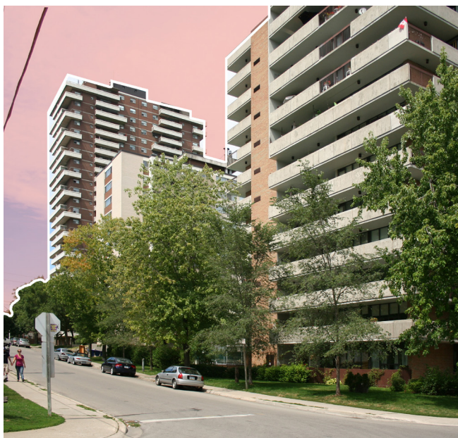
Figure 45: Residential Neighbourhood Mississauga, High St E and Helene St N, Image Credit: Google Map
