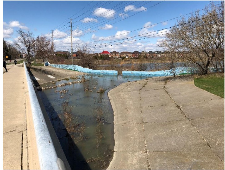
Plate 10: Channelization and culvert; disturbed, no potential
