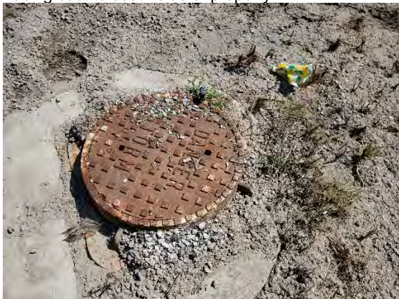
Storm sewer catchbasin
