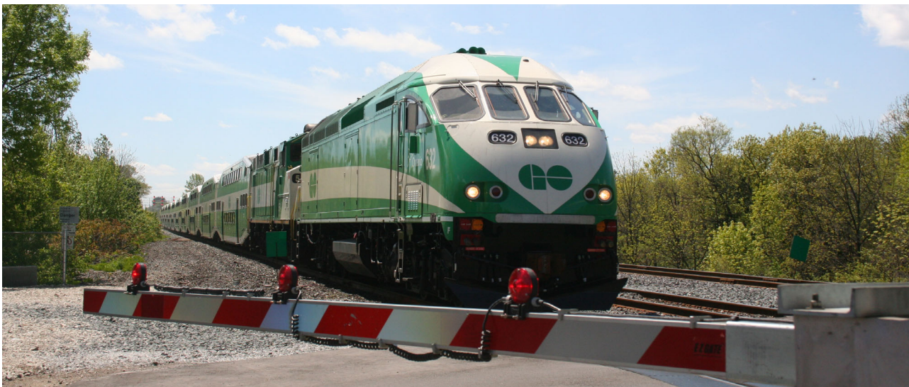
Figure 8-11: The rail corridors in Mississauga are shared by both freight and passenger trains, such as the GO train depicted above. The City recognizes these corridors as assets in the transportation system.
