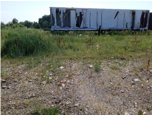
Plate 11: Construction debris on surface of soil in area of demolished shed at 5080 Ninth Line (facing east).
