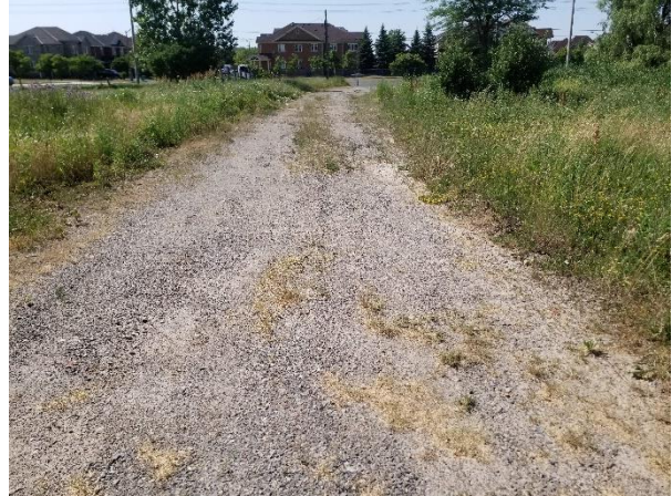
Plate 8: Gravel driveway at 5080 Ninth Line (facing northeast).
