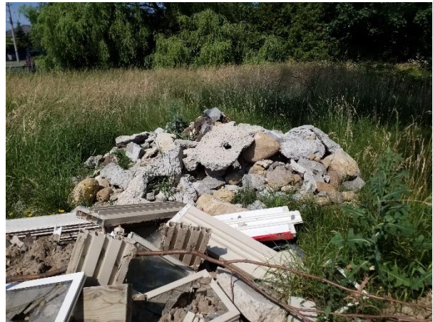
Plate 10: Debris from the demolished structure at 5080 Ninth Line (facing north).
