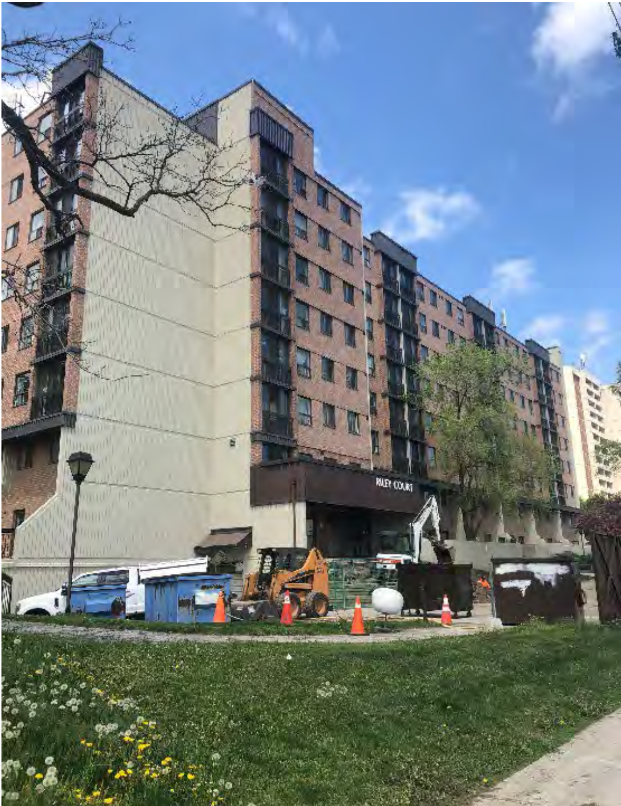
Figure 9-Existing 8 storey apartment building at 888 Riley Court
