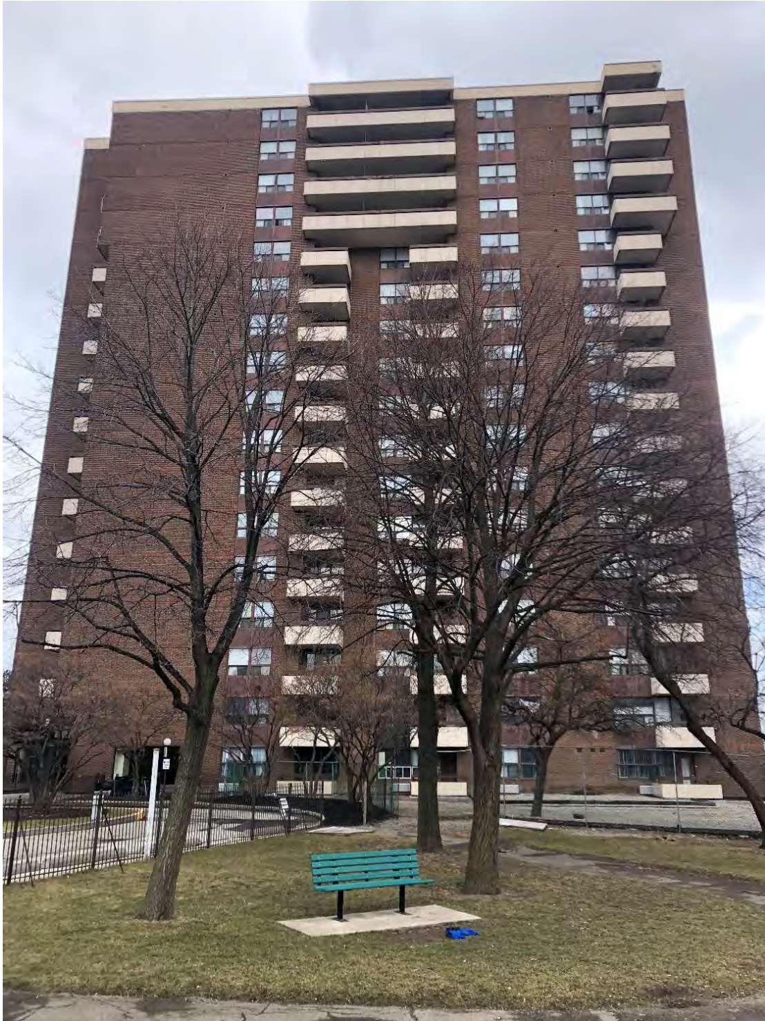
Figure 62- Existing 17 storey rental apartment building located at 600 Lolita Gardens
