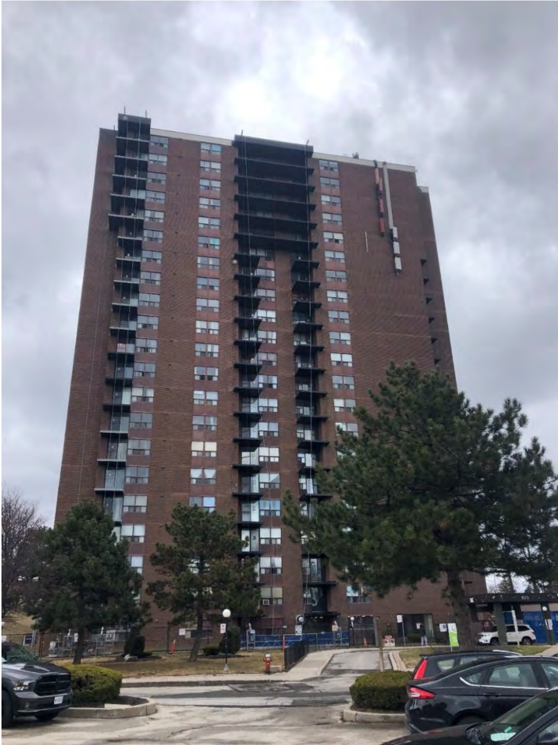
Figure 61- Existing 21 storey rental apartment building located at 620 Lolita Gardens
