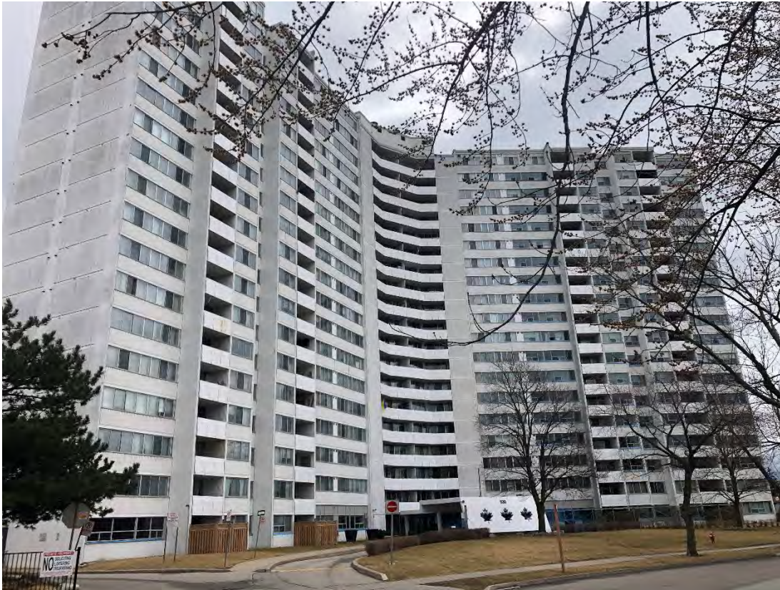
Figure 66- Existing 19 storey Apartment Building located at 530 Lolita Gardens
