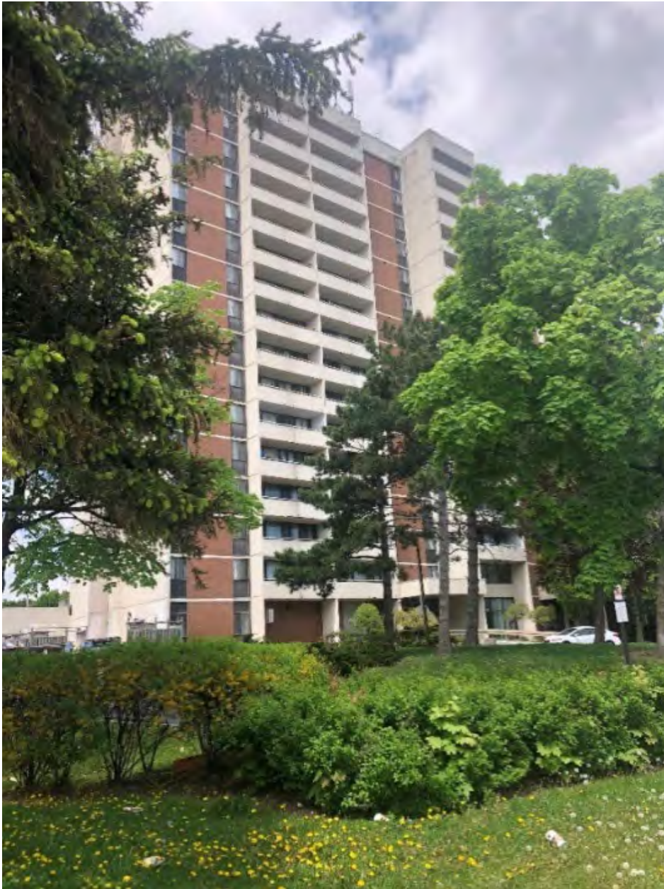
Figure 8-Existing 16 storey rental apartment building is located at 935 Dundas Street East
