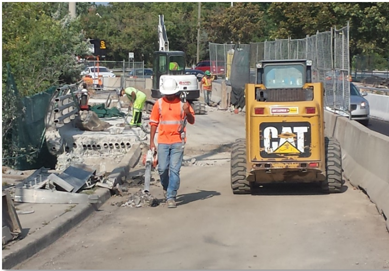
Bridge reconstruction on Burnhamthorpe Road over Sawmill Creek
