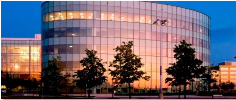
Mississauga Airport Corporate Centre
