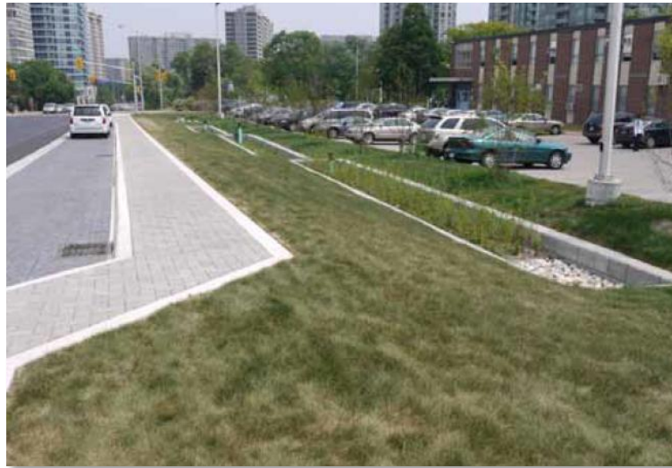
Bioswales at the Elm Drive Low Impact Development project
