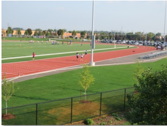
Loyola Secondary School Artificial Field, built in partnership with the Dufferin Peel Catholic District School Board
