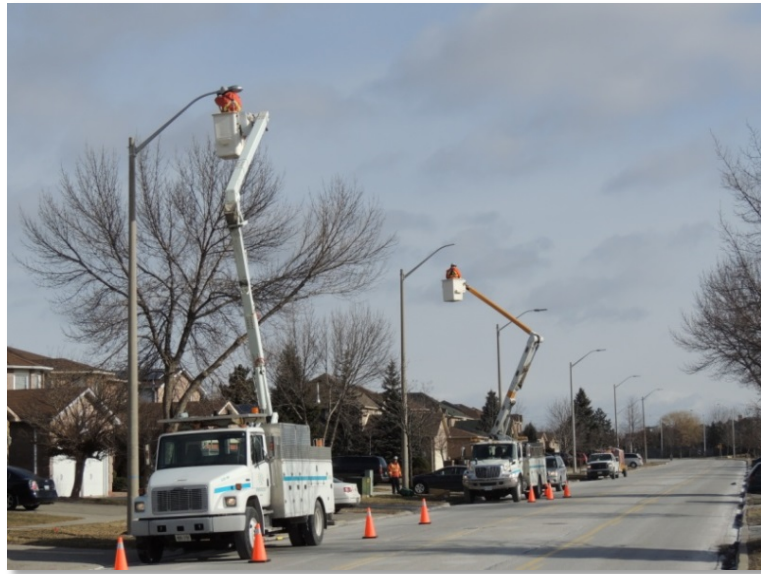
Over 80 per cent of streetlights have been upgraded to energy efficient Low Emitting Diode (LED) technology
