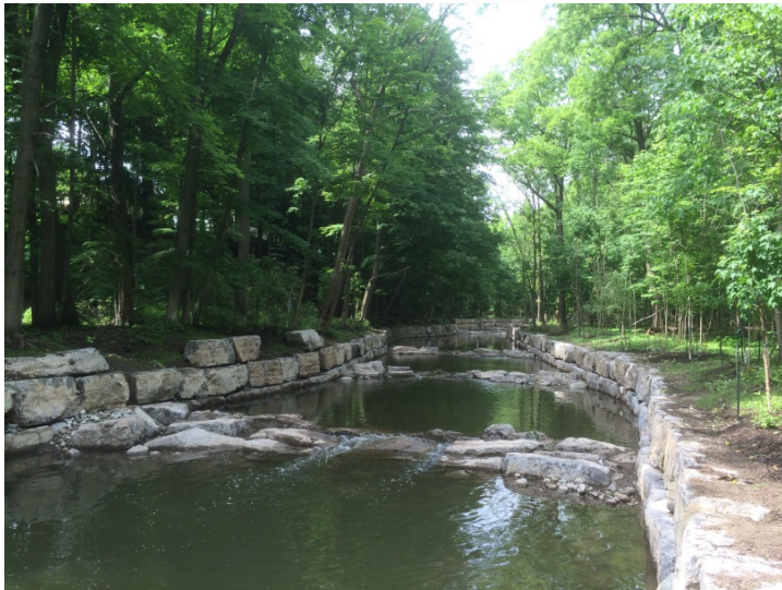
Creek erosion control bank stabilization at Sheridan Creek
