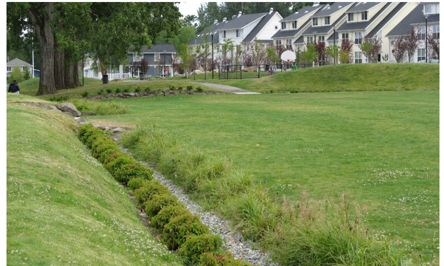
Figure 2.4a - Several LID practices are recommended to be implemented in the development, including enhanced grass swales or bioretention areas within parks and open spaces.
