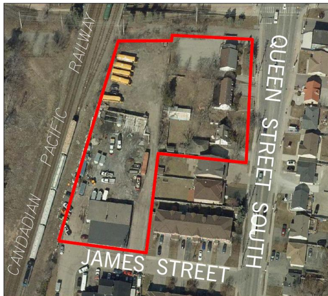
Aerial Photo of 6, 10, 12 Queen Street South, 16 James Street and 2 William Street
