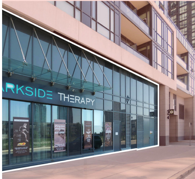
Figure 29: Transformer vault should be integrated into the design of buildings. Downtown Mississauga, Curran Place & Brickstone Mews
