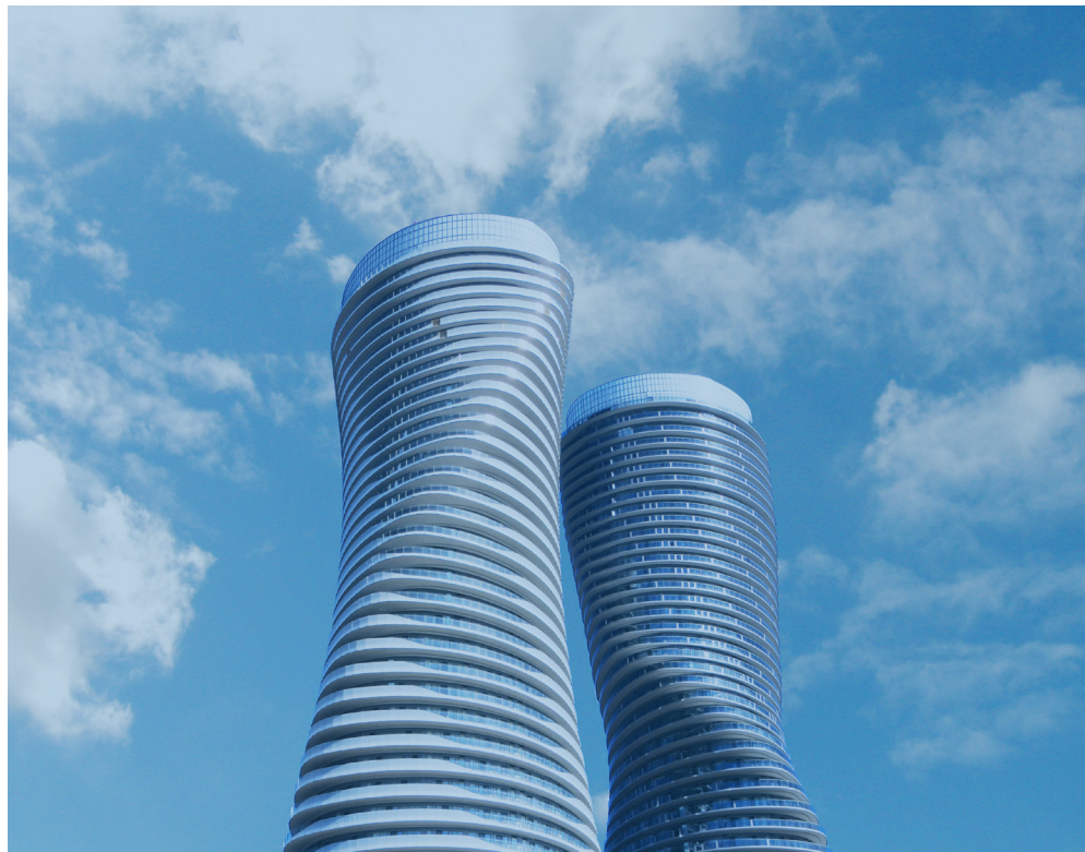
Figure 40: Absolute World is a residential condominium twin tower skyscraper complex. Downtown Mississauga, Hurontario St & Burnhamthorpe Rd E
