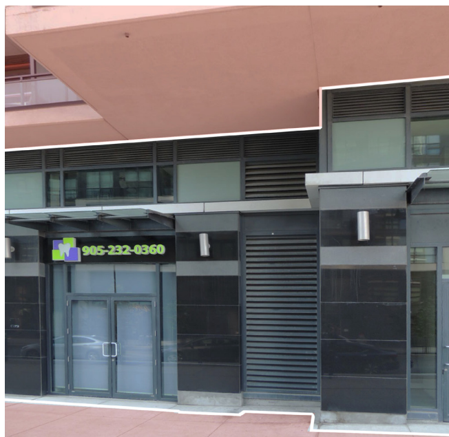
Figure 30: At grade exhaust vents serving structured parking facilities should be integrated into the design of buildings. Downtown Mississauga, Curran Place & Brickstone Mews
