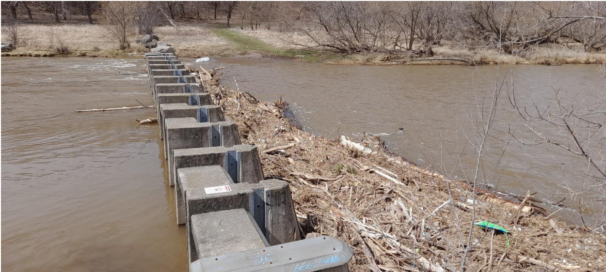
Plate 7: View of the ice control structure (A.S.I., 2023)
