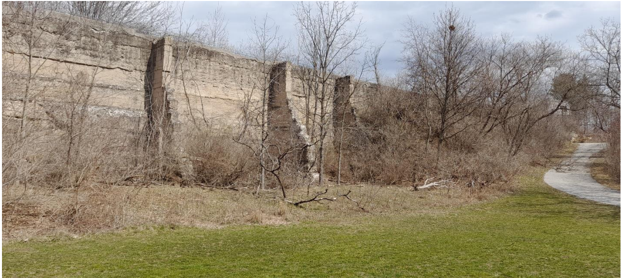
Plate 9: Remains of the Erindale Dam in the park (A.S.I., 2023)
