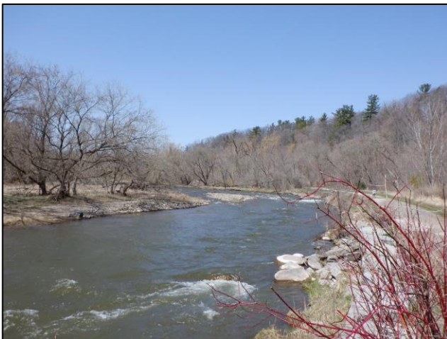
Figure 3-14: Armourstone Lined Bank through Reach CRED-0800
