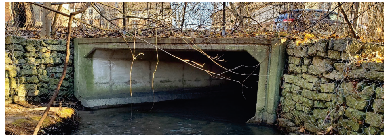
Example of Enclosed Watercourse in Storm Sewer
