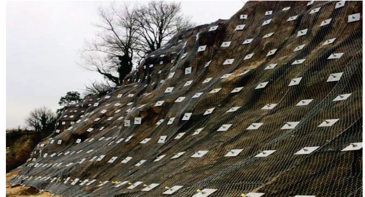
Example of Structural Bank Protection – Soil Nails
