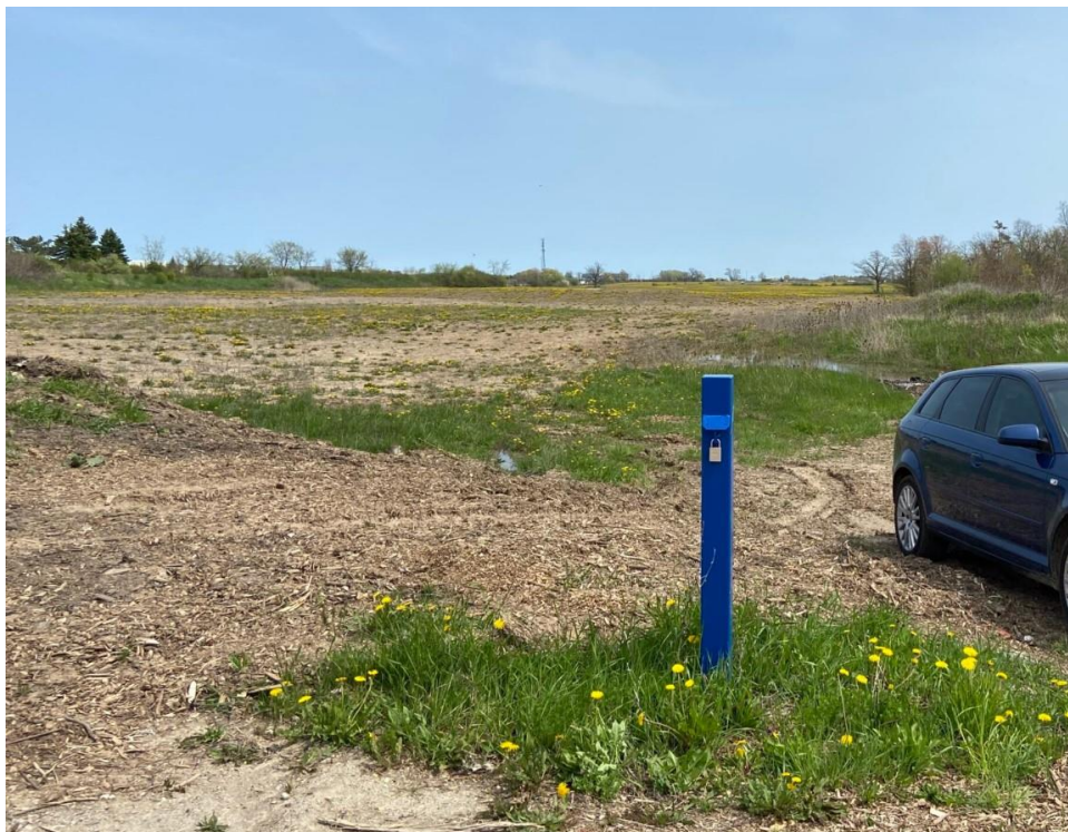
Photo 14: Looking south toward monitoring well MW8 installed near the south boundary.
