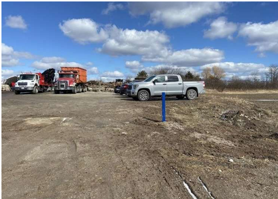
Photo 18: Looking north at groundwater monitoring well MW8 installed at BH8.
