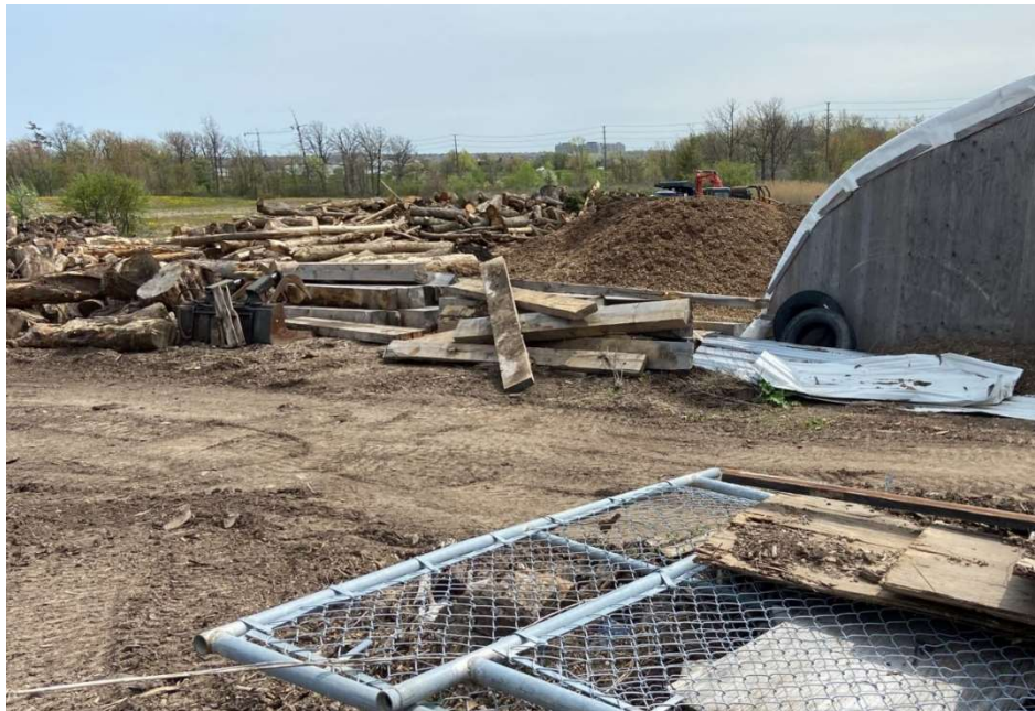
Photo 2: Wood and fence behind the storage shelter (Quonset hut) in the south part of the Site.
