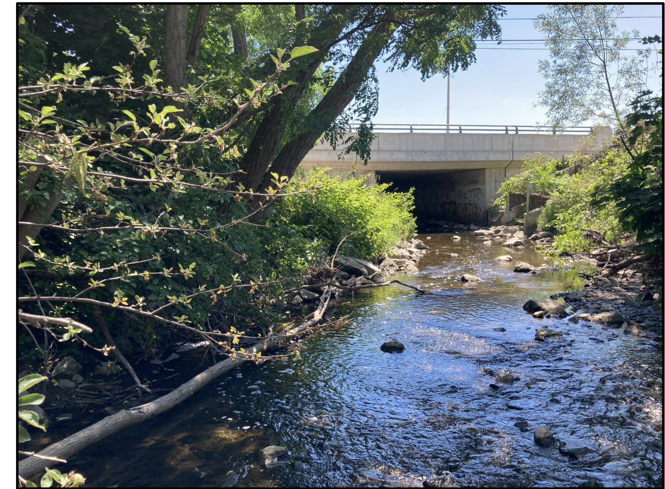
Dundas Street East Bridge (Matrix 2021)
