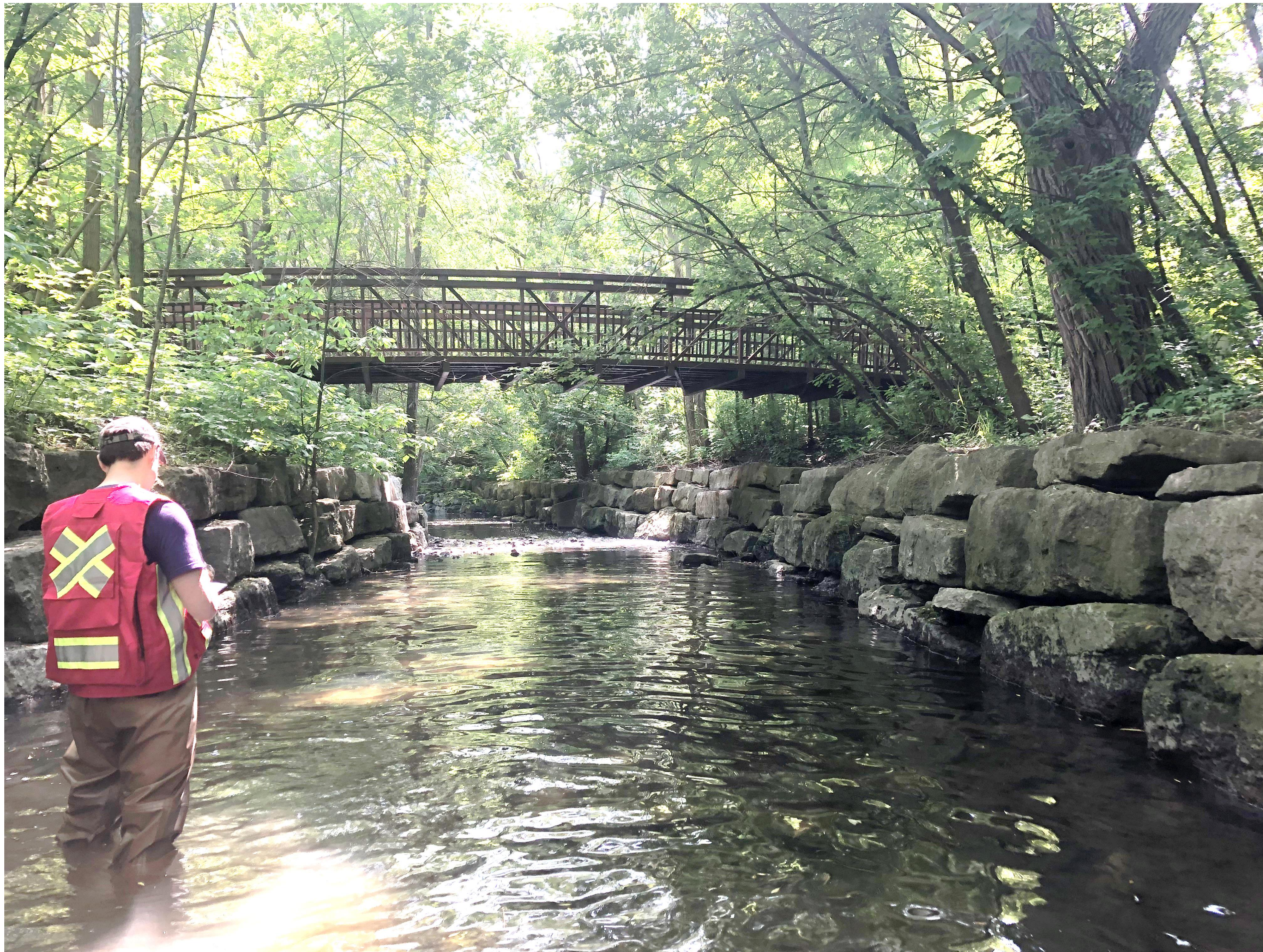
Upstream of Dixie Road
