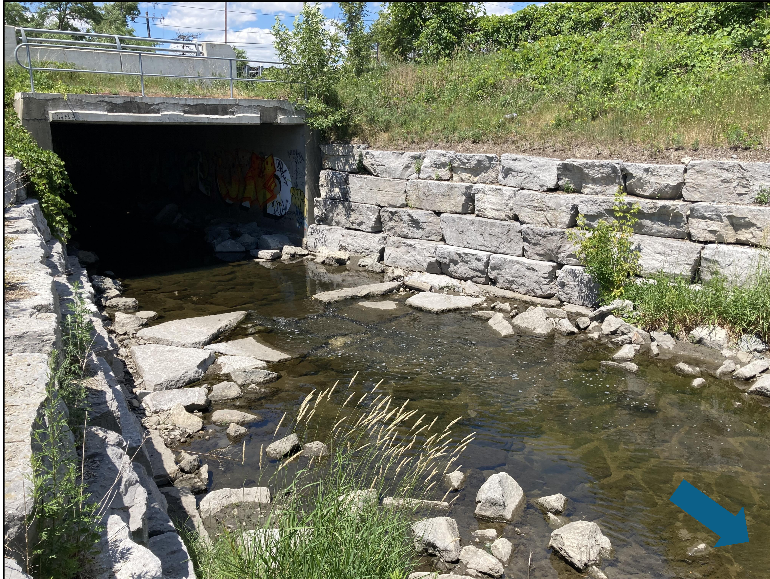
Existing Dundas Street East Crossing (Matrix 2021)
