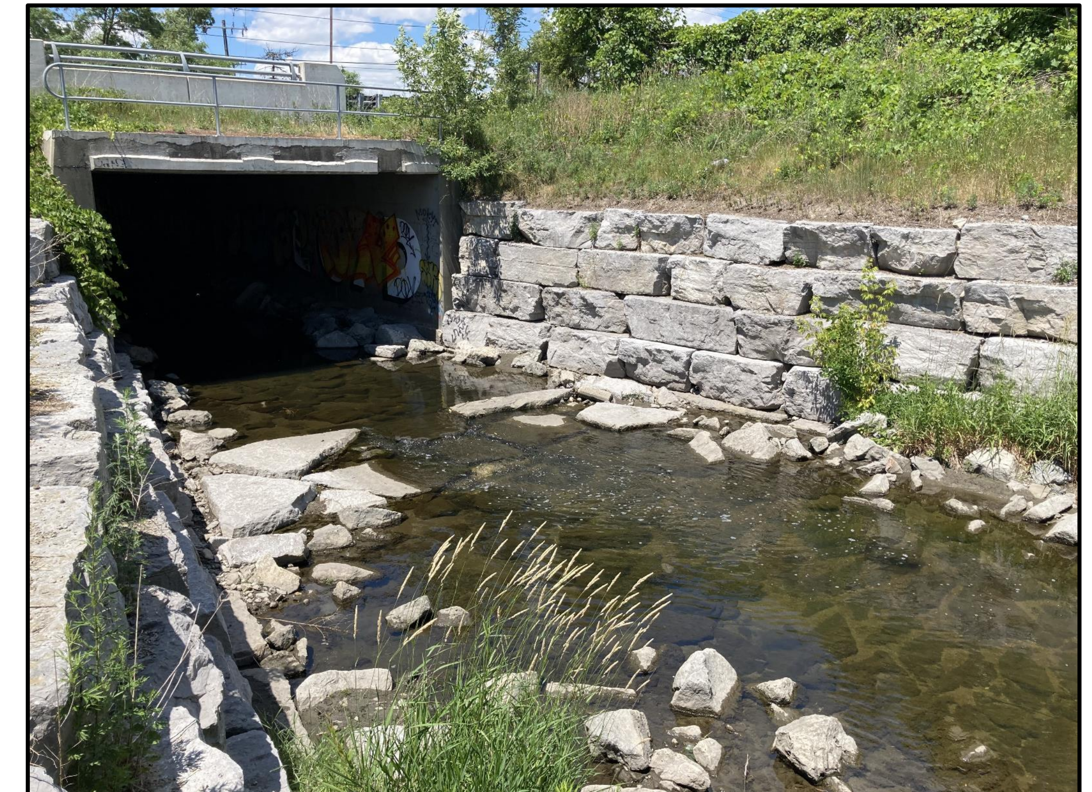
Existing Dundas Street East Crossing (Matrix 2021)
