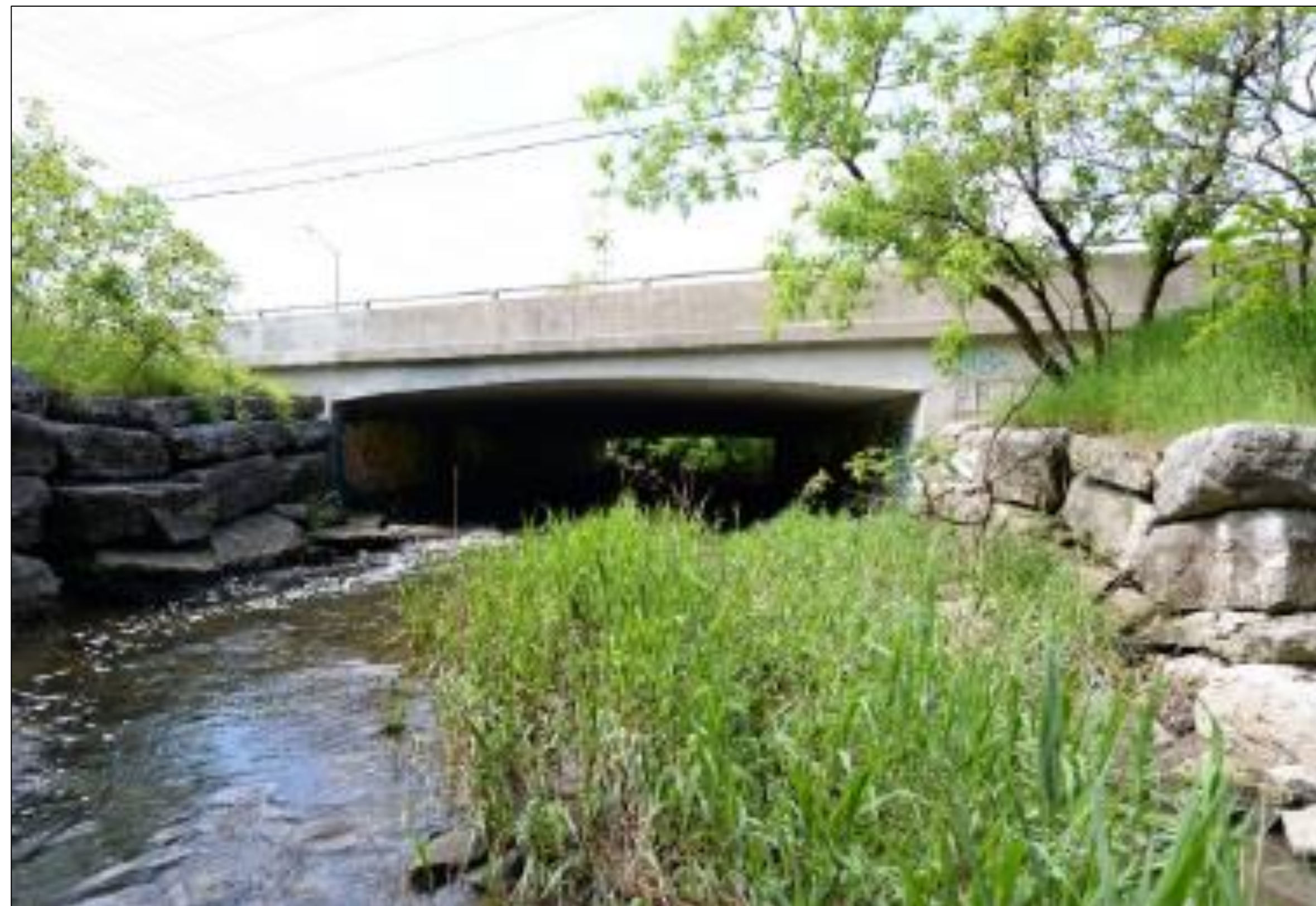
12 m span Dixie Road Bridge (Thurber 2019)
