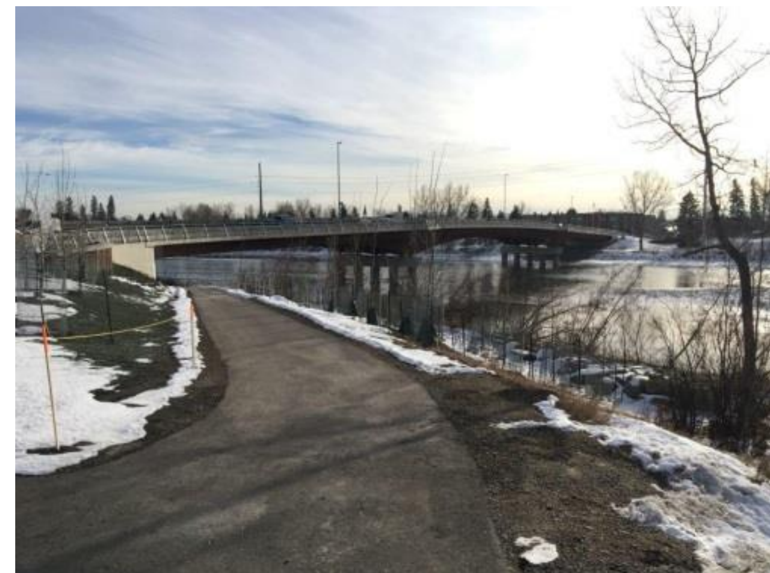
Double Span Bridge
