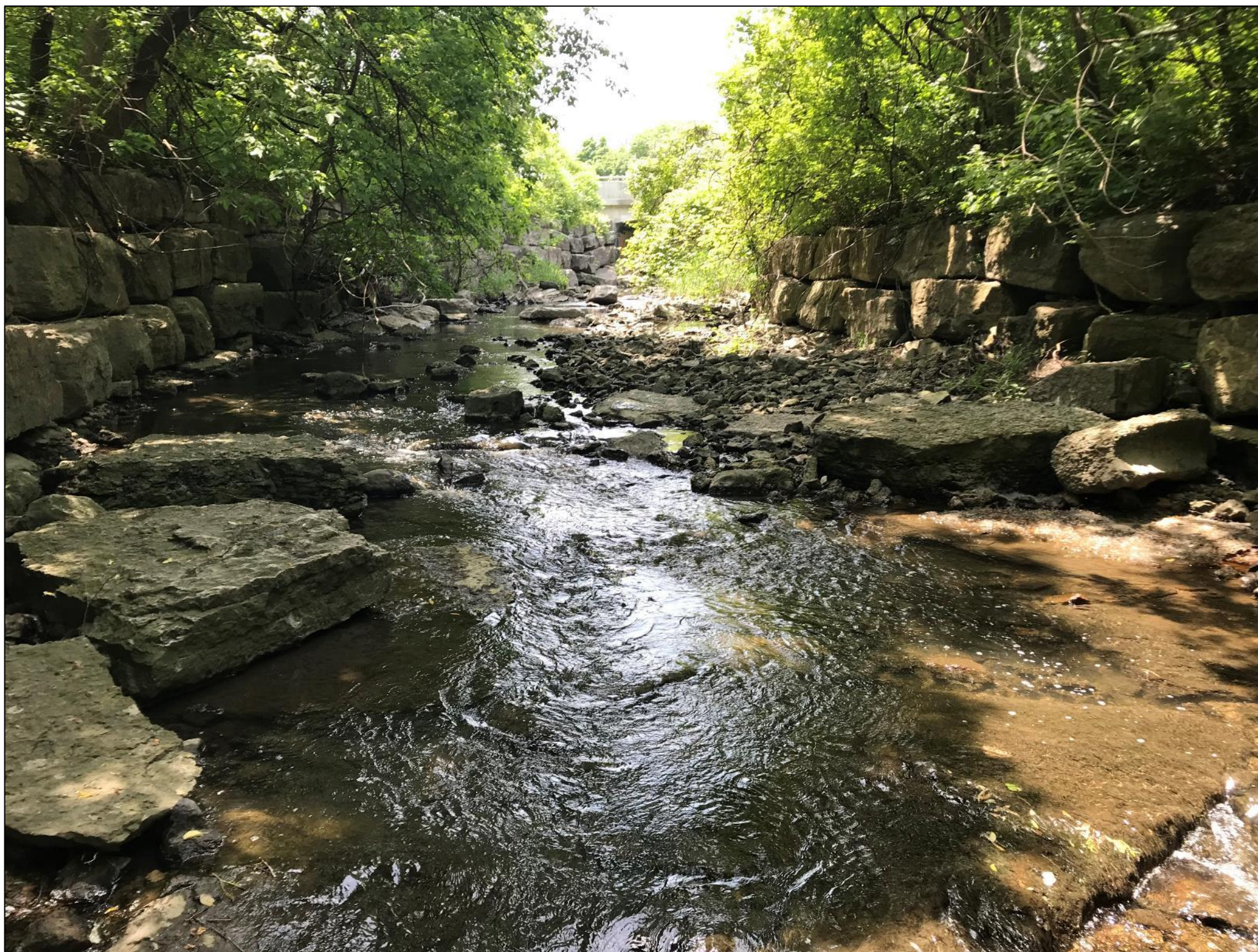
Downstream of Dixie Road (Matrix 2019)
