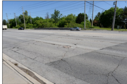
Dixie Road Bridge (Thurber 2019)
