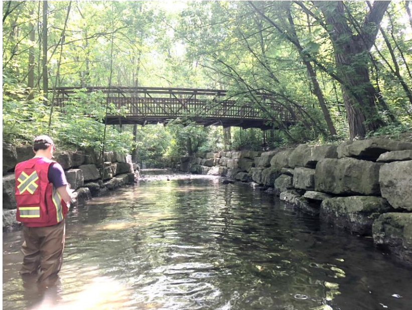
Upstream of Dixie Road
