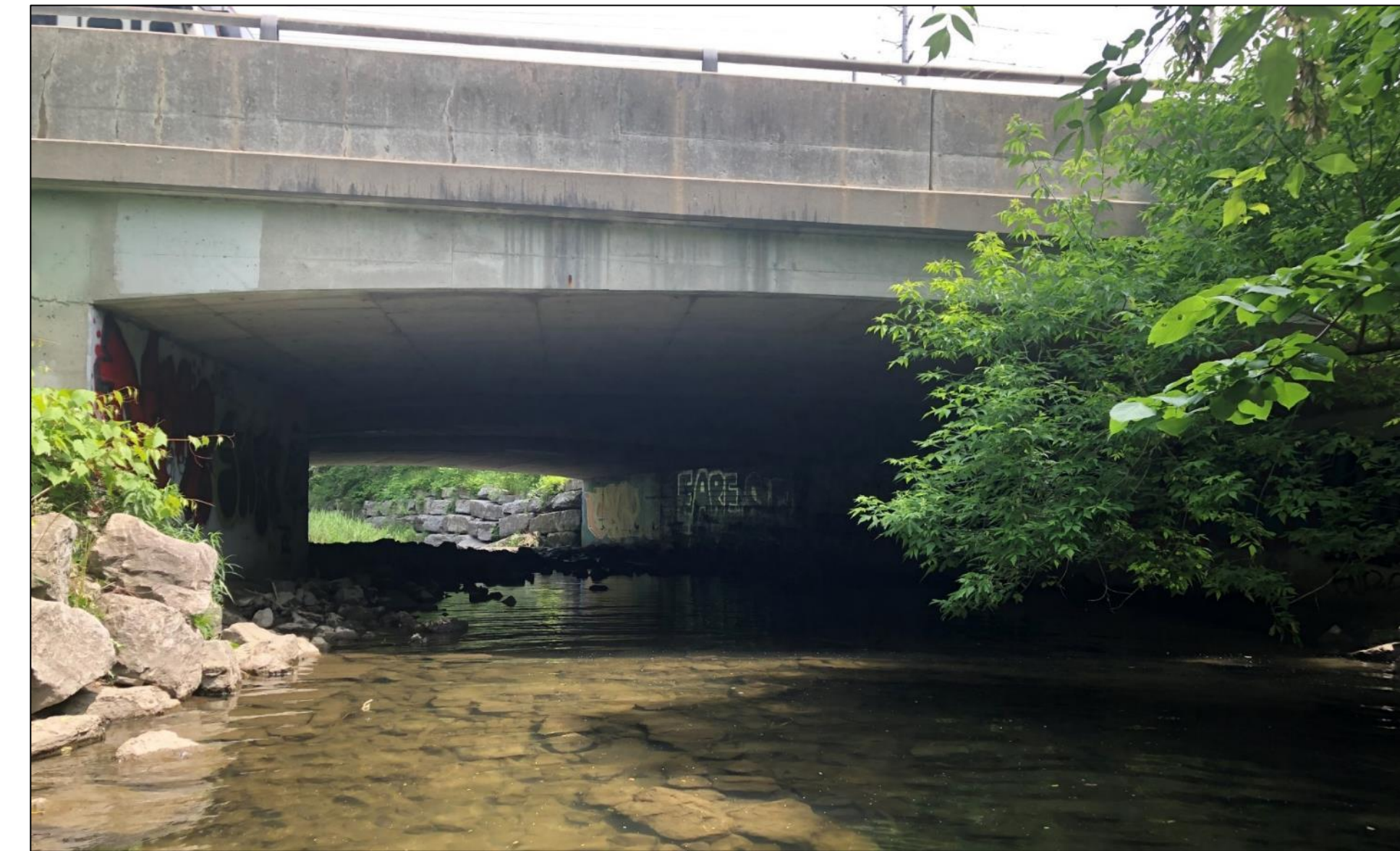
Dixie Road Bridge
