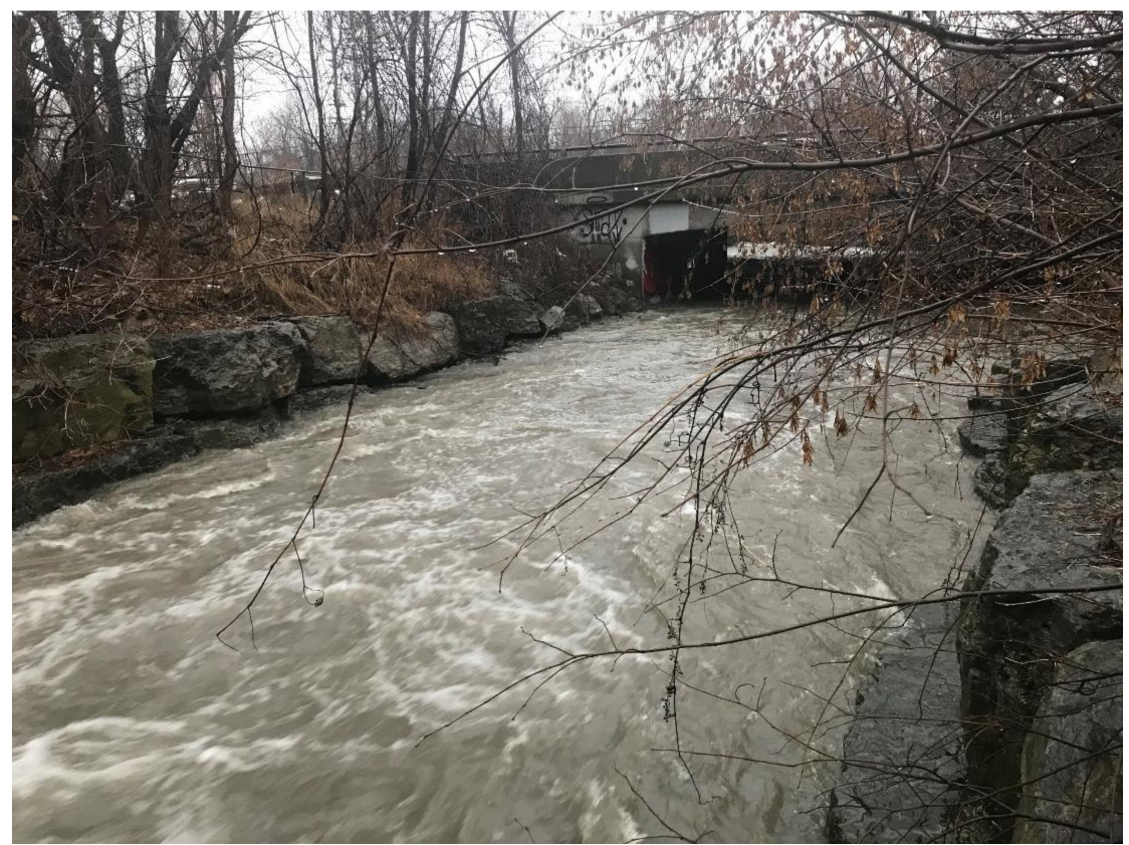
Dixie Road Bridge Crossing (Matrix 2020)
