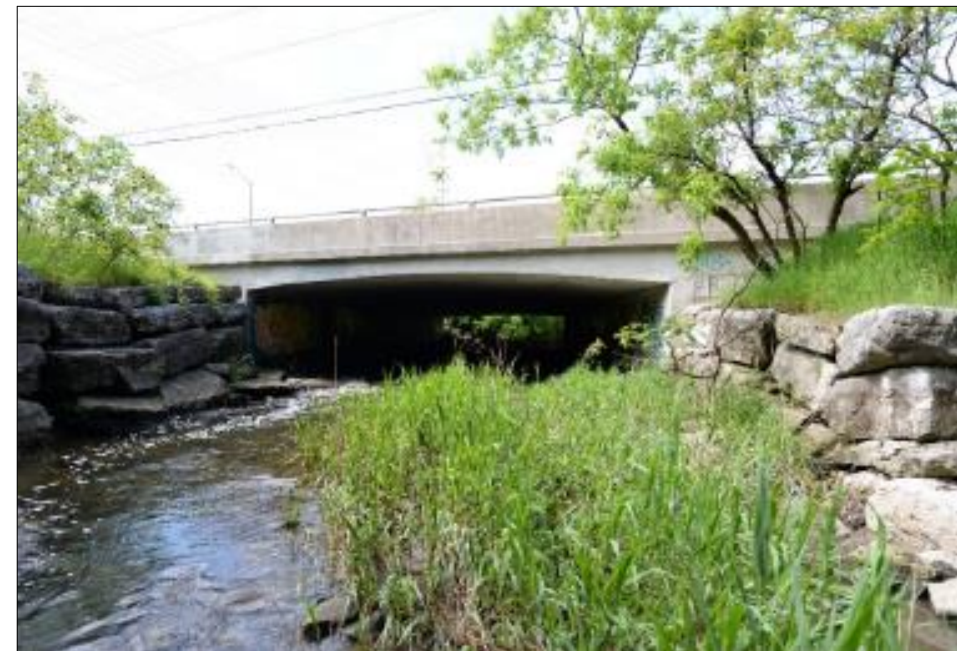
12 m span Dixie Road Bridge (Thurber 2019)
