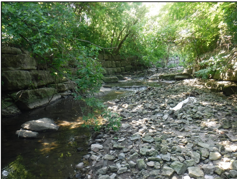
10. Channel has larger areas of deposition directly downstream of Dixie Road which has created areas of concentrated flows.
