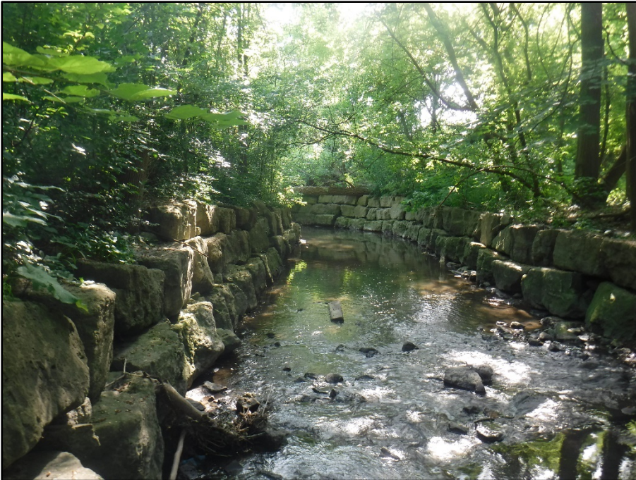
5. The channel continues to be heavily armored moving downstream towards Dixie Road.
