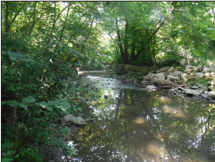
2. Channel armoring changes from large boulders to armour stone along the banks.
