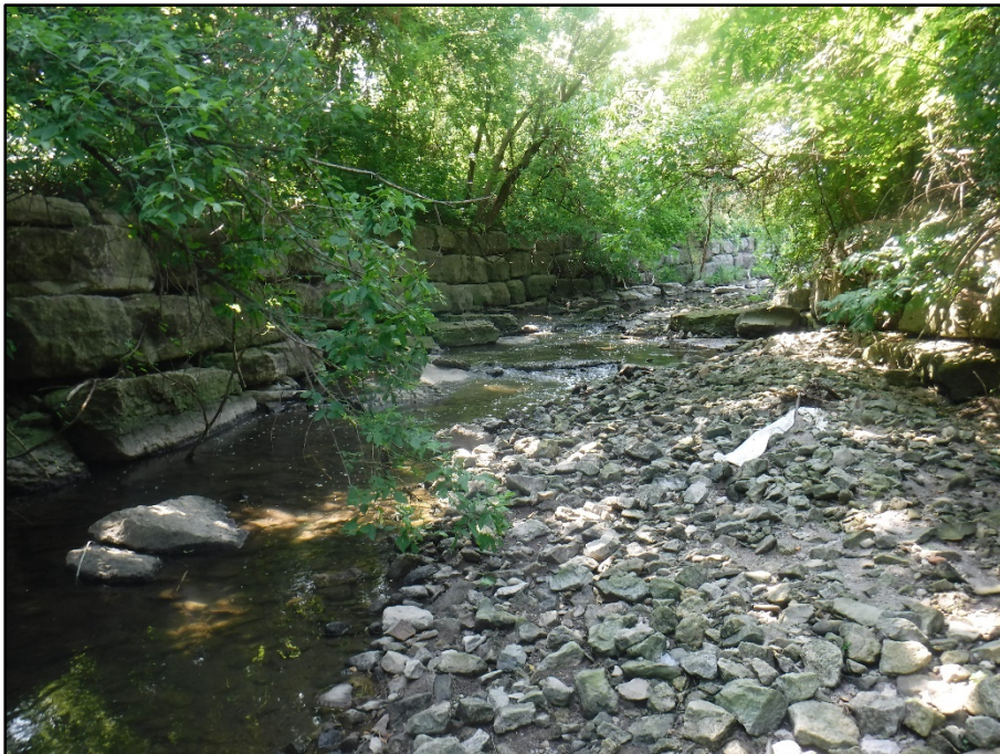
14. Channel has larger areas of deposition directly downstream of Dixie Road which has created areas of concentrated flows.
