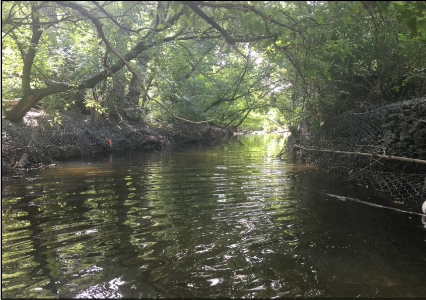
19. Gabion baskets create a slow flowing pooled habitat with overhanging vegetation.
