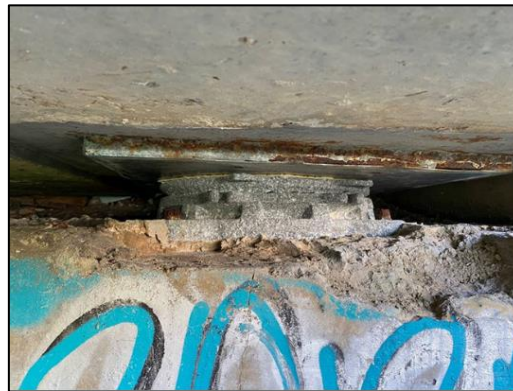
Removed Loose Concrete and Salt
