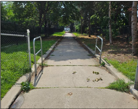
Example Engineered Walkway
