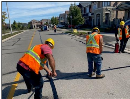
Crack Sealing Repairs and Road Rehabilitation
