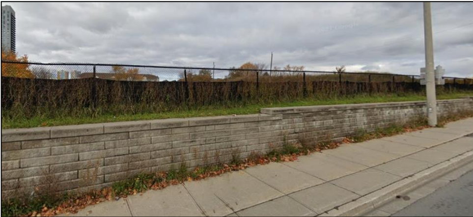
Example Retaining Wall
