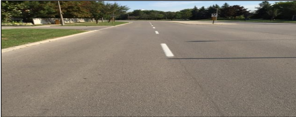
Example of Road Pavement in Very Good Condition
