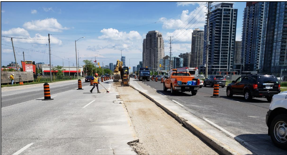
Hurontario median removals for LRT
