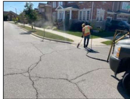
Crack Sealing Repairs and Road Rehabilitation
