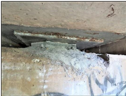
Power Washing of Bearing Seats on Burnhamthorpe Road West Structures
