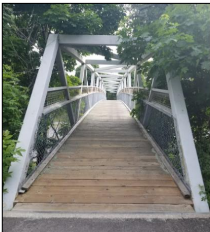
Example Pedestrian Bridge
