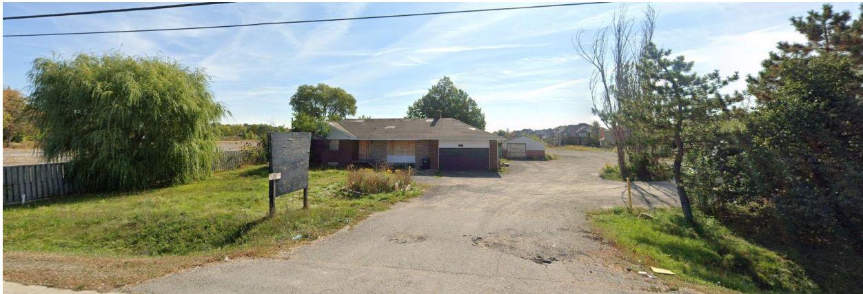
Photo of Existing Site Condition (view south from Derry Road West)
