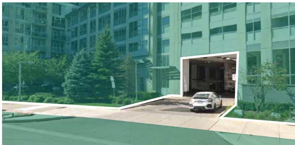
Figure 22: Provision for vehicular access to off-street parking, access for deliveries, garbage pick-up, servicing and loading.
