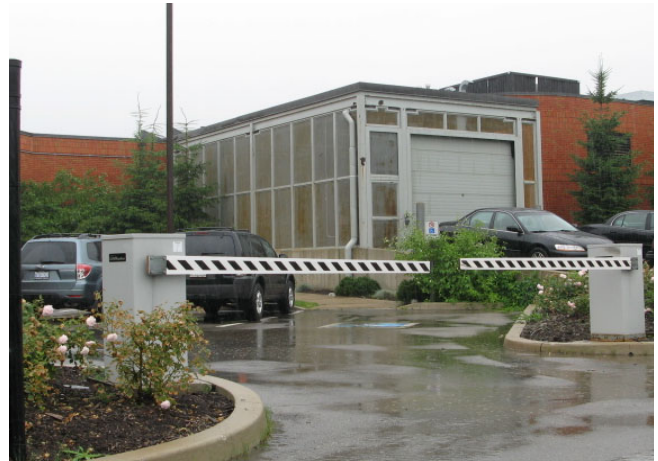
Figure 3.4.1 Mechanical security control
