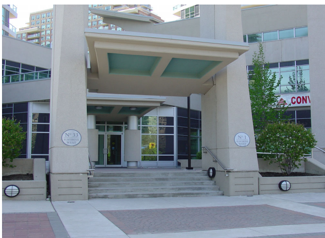
Figure 4.2.1 Columns & canopy provide spatial definition to the lobby entrance
