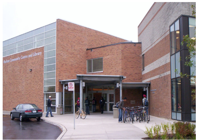
Figure 4.3.2 After —The removal of pergola & bringing the entranceway forward increases visibility from the parking lot & street
