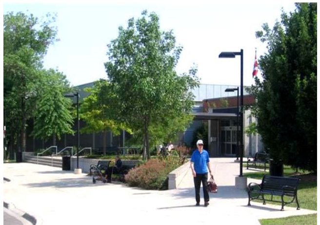
Figure 3.0.2 A Community centre entrance which incorporates accessibility & safety into the design
