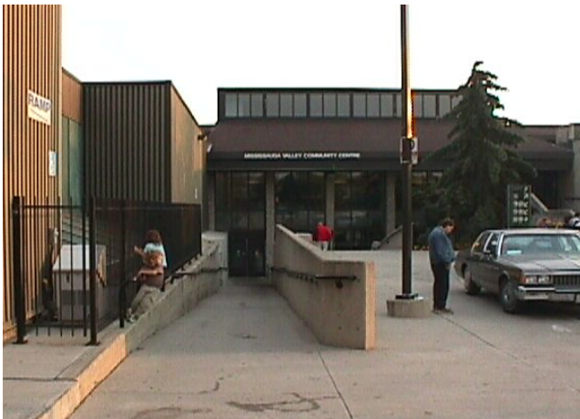
Figure 4.0.1 Before—Mississauga Valley Community Centre with sunken entranceway which results in poor visibility
