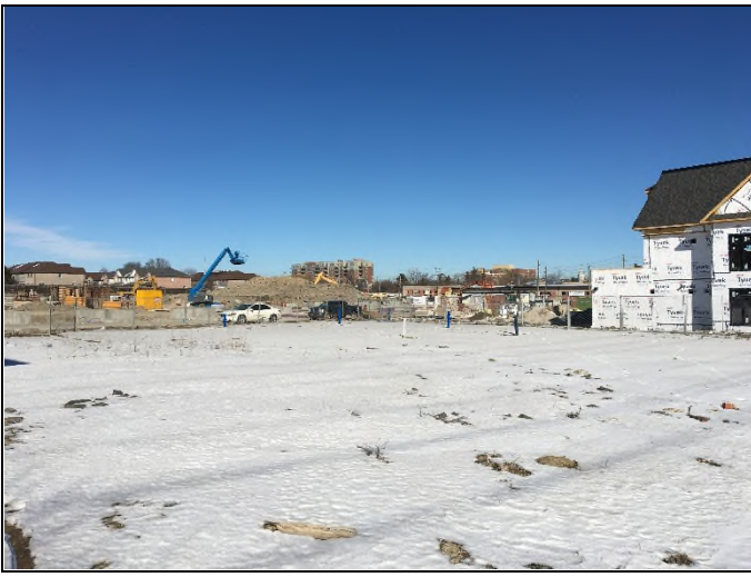
1. 86 Thomas Street – View of the Site looking northeast.
