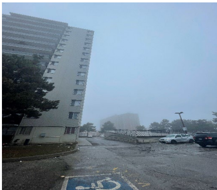
Photo #11: Southeast portion of 1850 Bloor Street, facing north.
