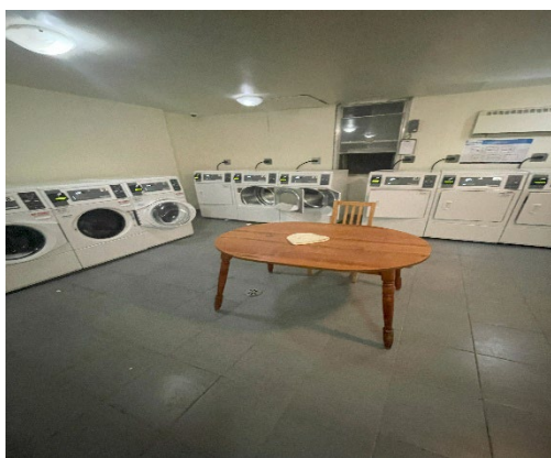
Photo #29: Laundry room located in the basement of 1850 Bloor Street.
