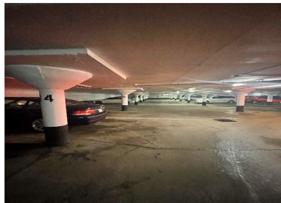
Photo #30: Underground parking area located in 1850 Bloor Street.
