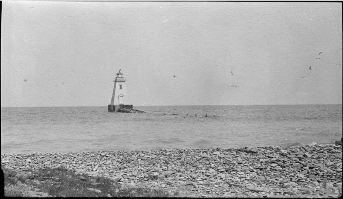
Figure 21: Pier Almost Fully Submerged 1917 (online MIKAN No. 3393405)
