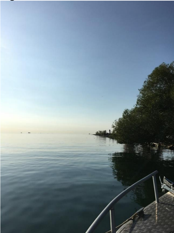
Figure 6: East Breakwater from North End facing South
