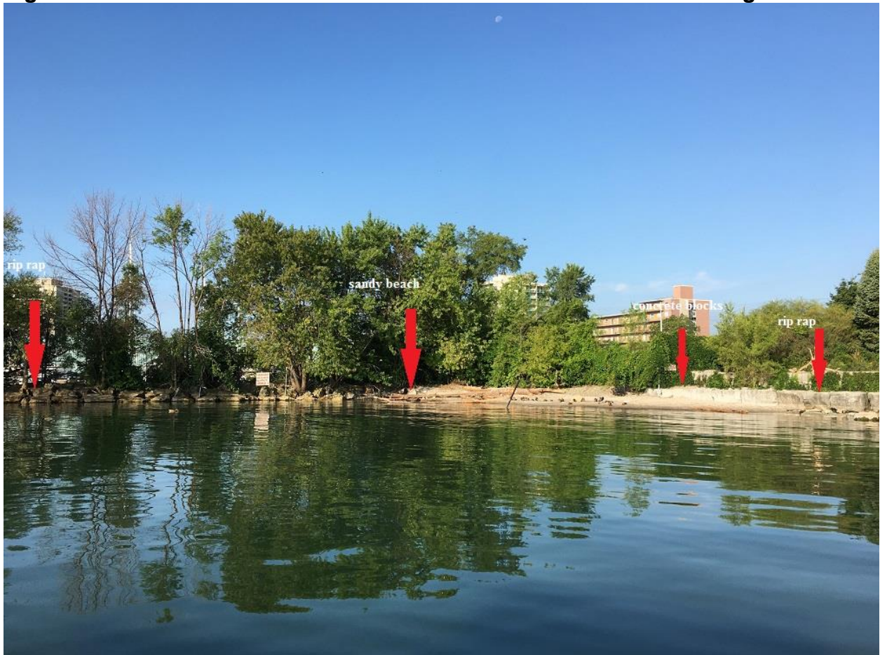
Figure 2: Modified Shoreline – Inside Corner of East Breakwater facing NW
