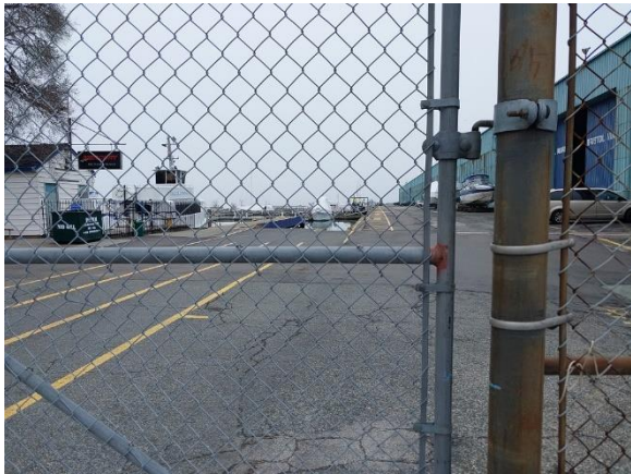
Image 8: Existing pavement facing SE
