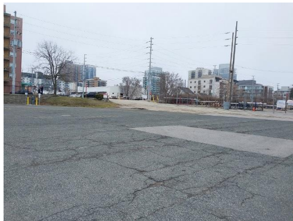
Image 5: Pavement facing north
