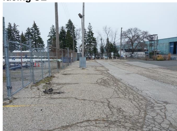
Image 24: Disturbed Area (paved) facing SE
