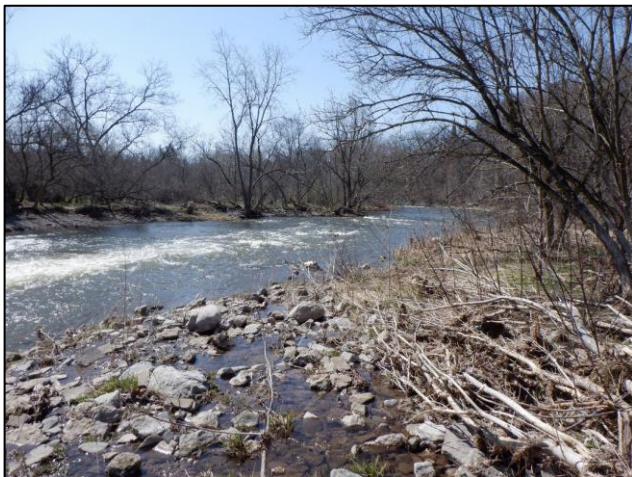
Figure 3-10: Reach CRED-0700 Downstream of the Ice Control Structure
