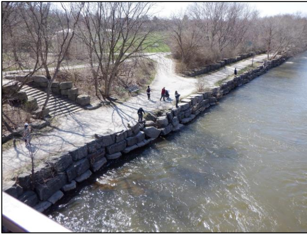
Figure 3-12: Armourstone Retaining Wall and Pedestrian Trail through Reach CRED-0700
