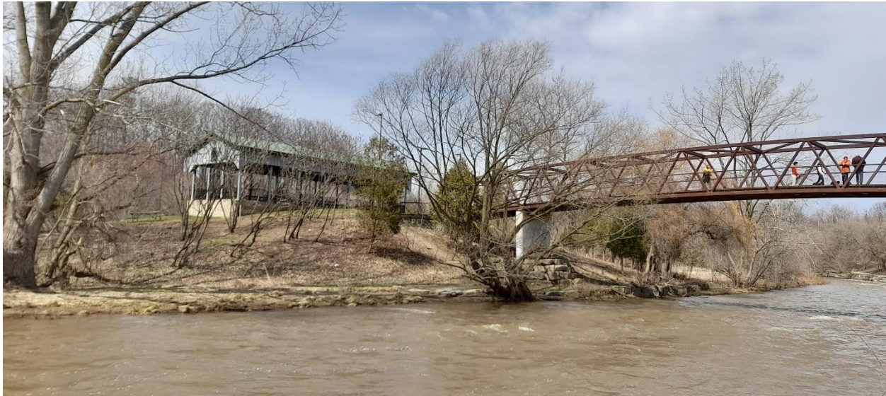
Plate 19: View of pedestrian bridge and covered picnic area within Erindale Park (A.S.I. 2023).
