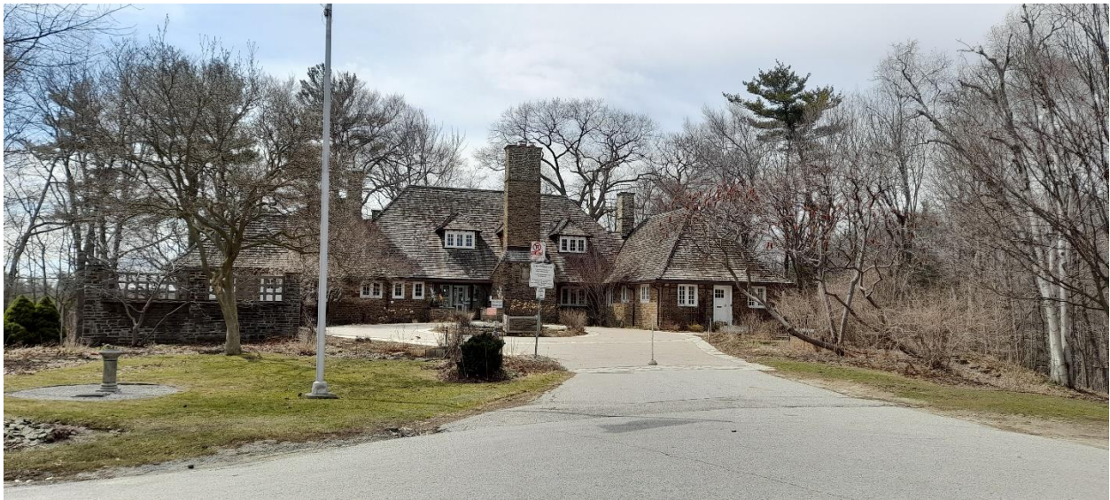
Plate 10: Chappell House, now the Riverwood Conservancy (A.S.I., 2023)
