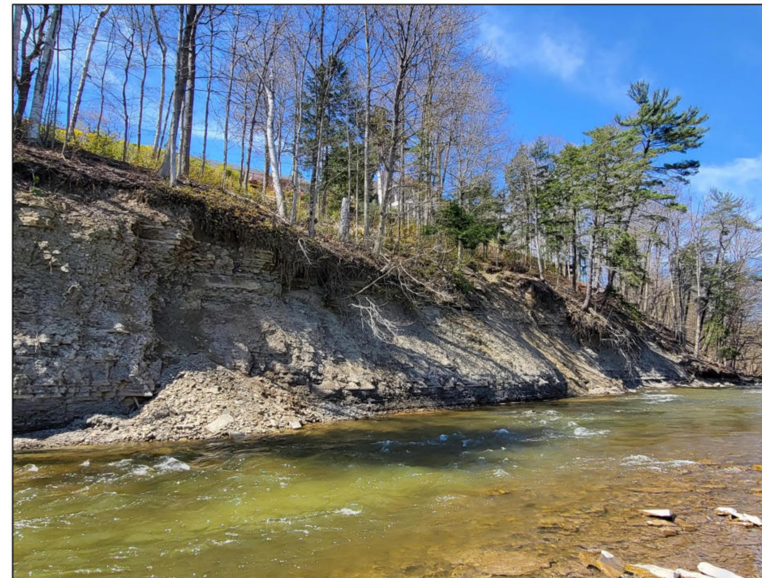
Valley Wall Erosion and Slope Instability
