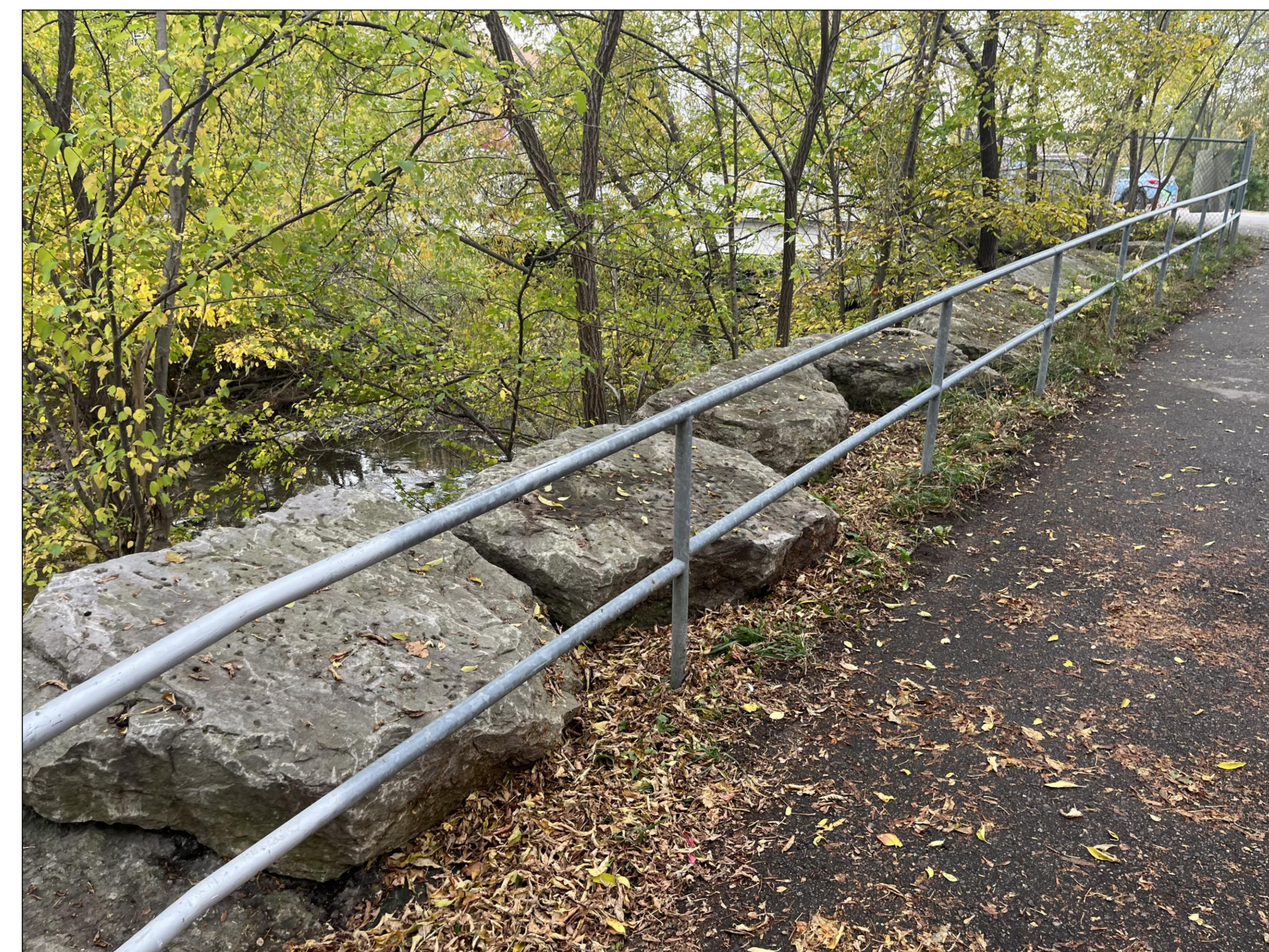
Armourstone Retaining Wall Along Trail
