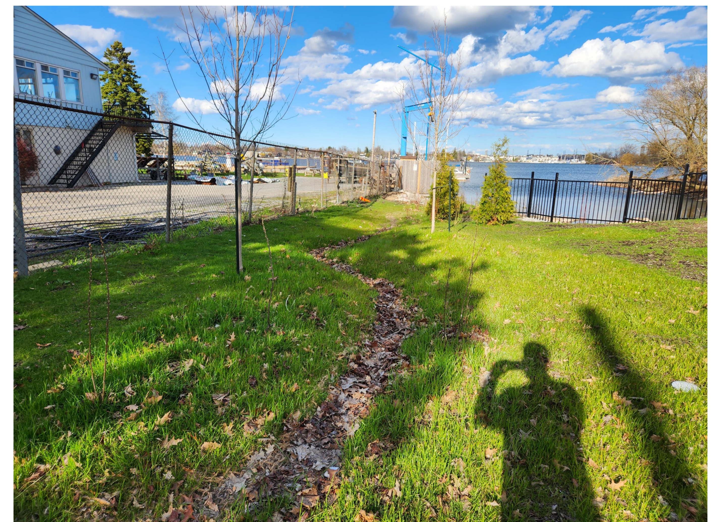
Example of Vegetated Drainage Swale
