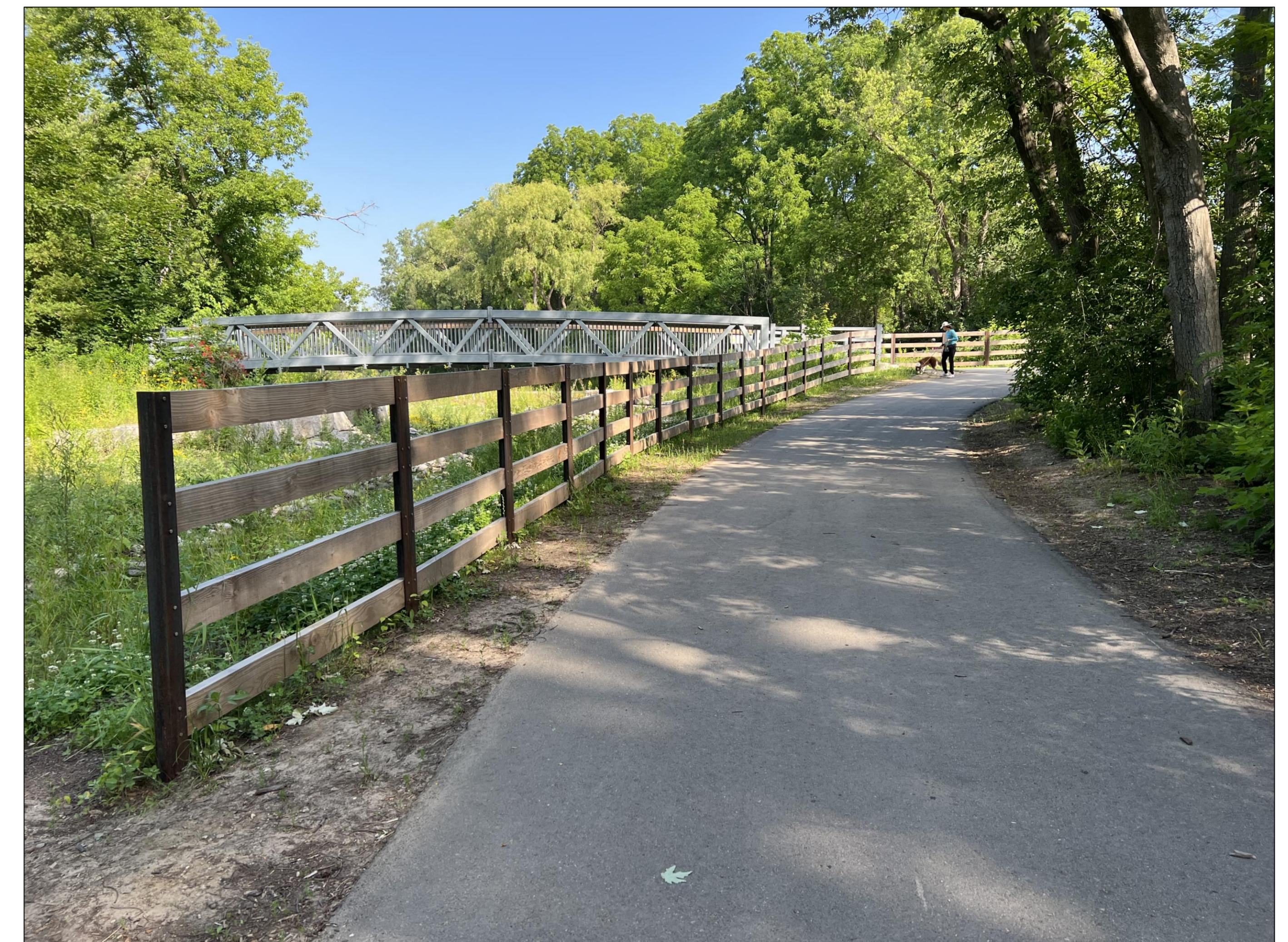
Example of Asphalt Trail Restoration with Safety Fencing
