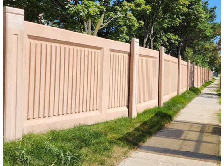
Mississauga Standard Concrete Noise Wall
