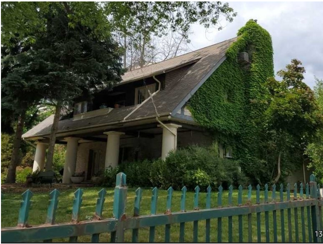
Photo 7: View of the Site Building B, Facing west.
