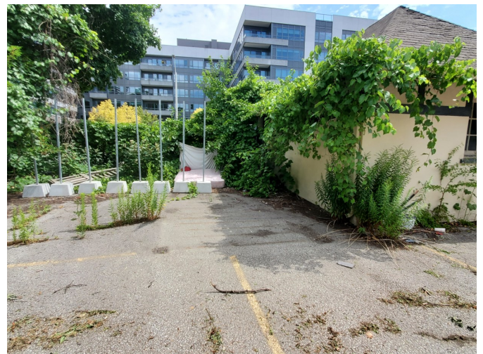
Photo 12: View of the square shaped storage shed (right), and the location of the former three (3) storage units, located north adjacent to the Site Building B.
