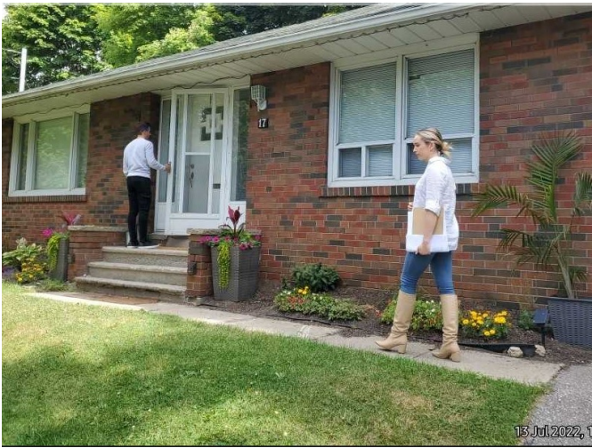
Photo 13: View of the west (front) portion of the Site Building C, Facing east.
