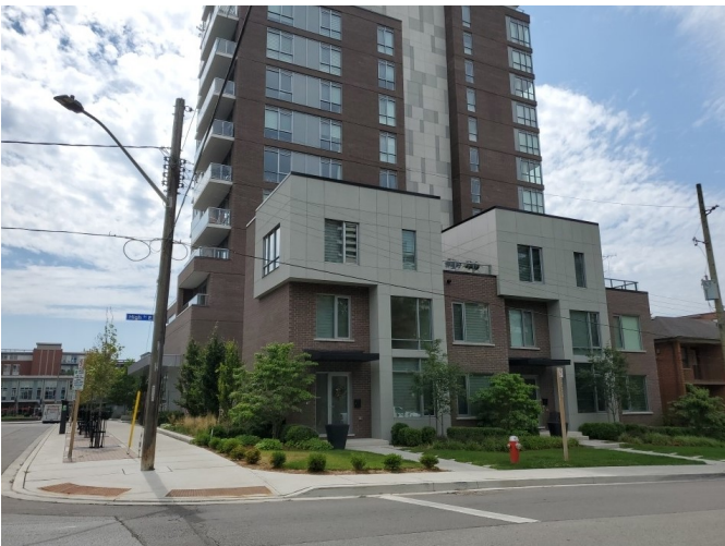
Photo 21: View of the adjacent residential high rise, southeast corner of Ann Street and High Street East, facing southeast.
