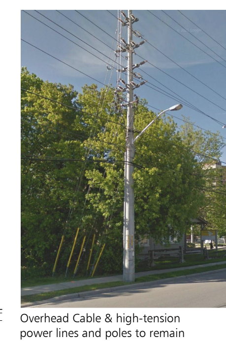
Overhead Cable & high-tension power lines and poles to remain
