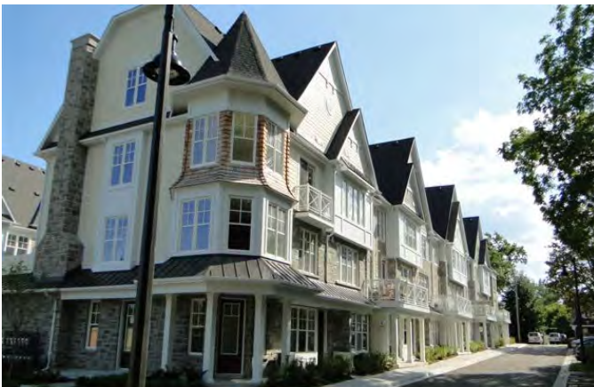
Figure B25 - Example of horizontal multiple dwelling in lakeview from an internal road
