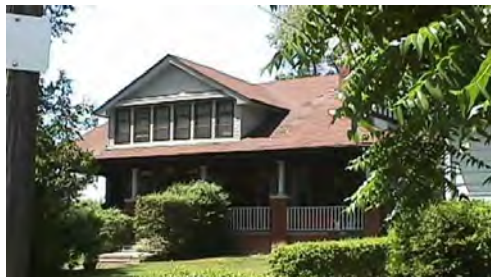
Figure B69 - Waseem Residence , 1273 St. James Avenue
