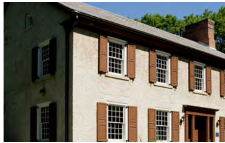
Figure B83 — Plaster
