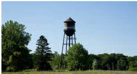
Figure B53 - Water Tower
