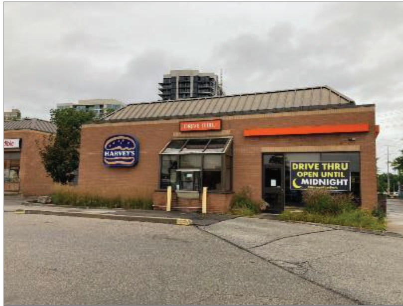
Photo 3 – Southwestern side of Site Building A.
