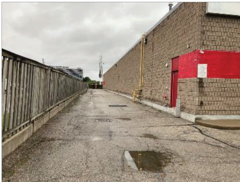
Photo 18 – Southwest side of Site Building D.
