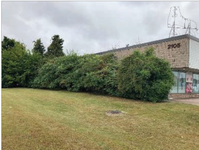
Photo 17 – Southeast side of Site Building D.
