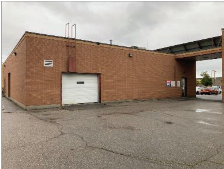
Photo 6 – Northwest side of Site Building B.
