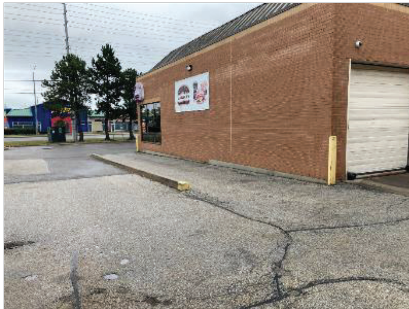
Photo 2 – Northeastern side of Site Building A.
