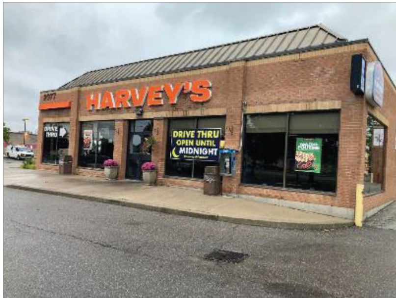
Photo 1 – Southeastern side of Site Building A, looking northwest.
