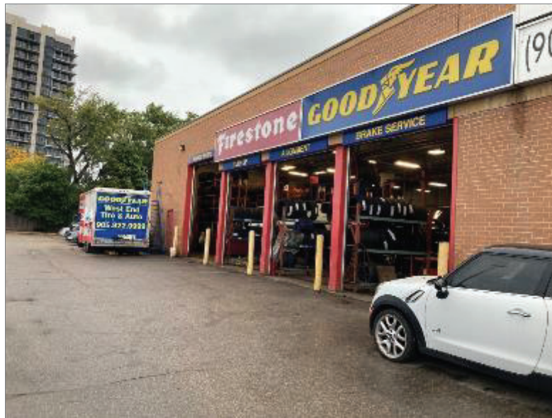
Photo 9 – Northwest side of Site Building C.
