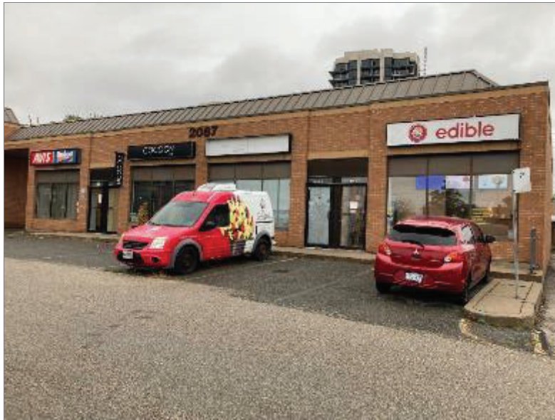
Photo 5 – Southwestern side of Site Building B.
