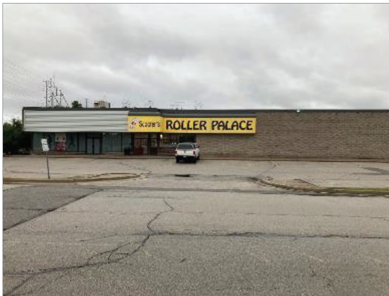
Photo 16 – Northeast side of Site Building D.
