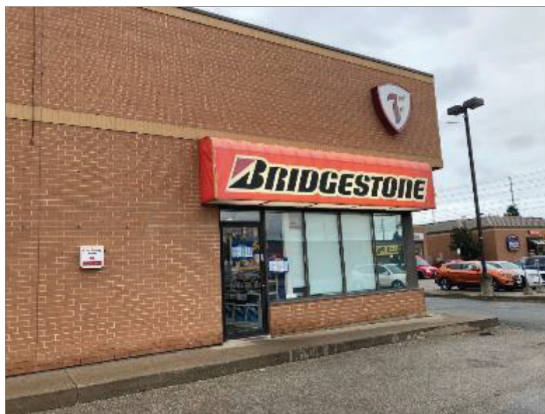
Photo 10 – Southwest side of Site Building C.
