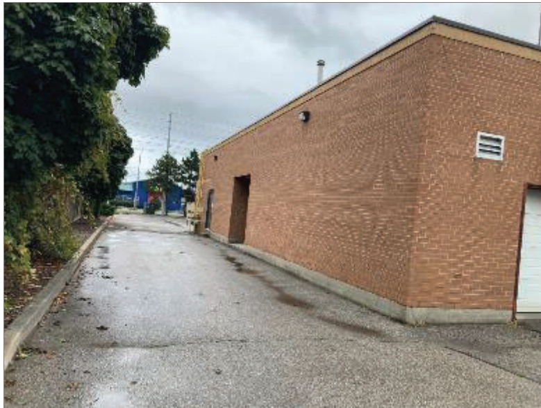
Photo 7 – Northeast side of Site Building B.
