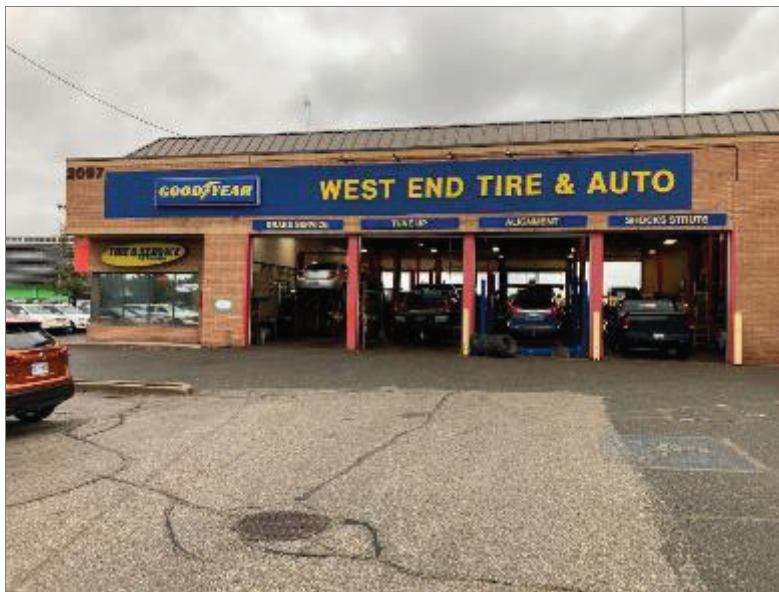
Photo 8 – Southeast side of Site Building C.
