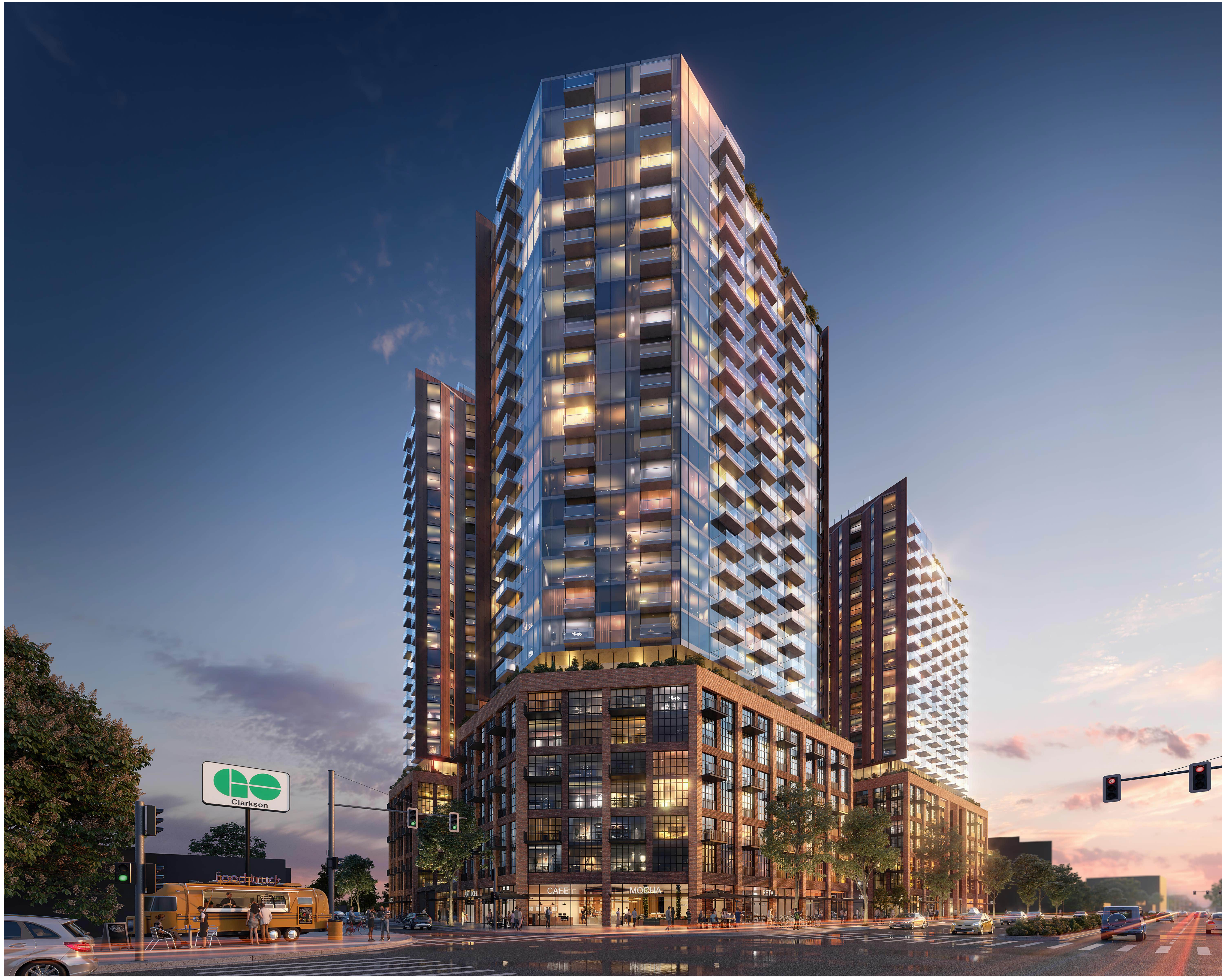
STREET LEVEL VIEW FROM SW CORNER
