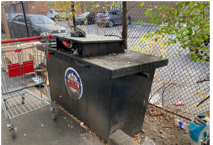
Photo 12: Grease bin for Al-Najmah Fine Foods supermarket located by garbage compactor and refrigerant compressors, facing southeast.
