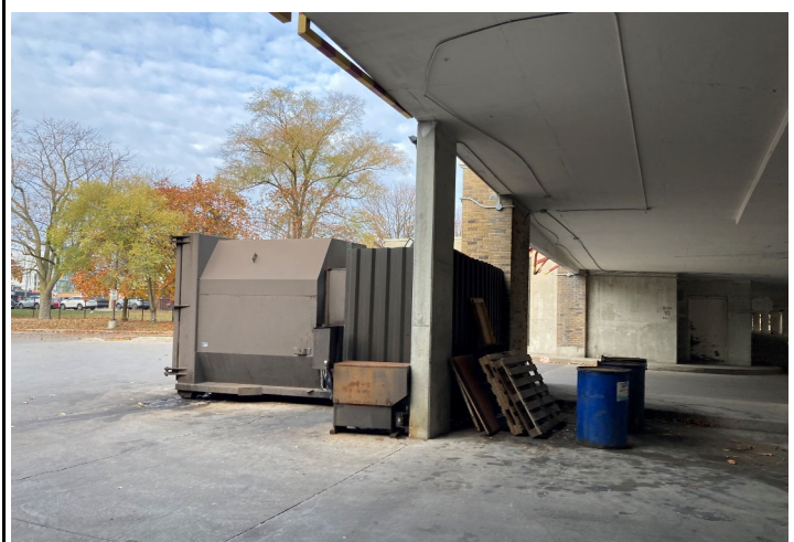
Photo 9: Garbage compactor and drums for used cooking oil located in concrete parking structure, facing west.
