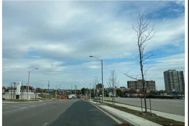
Photo 24: Parking lot for Oakville GO Station within Phase One Study Area, facing north.
