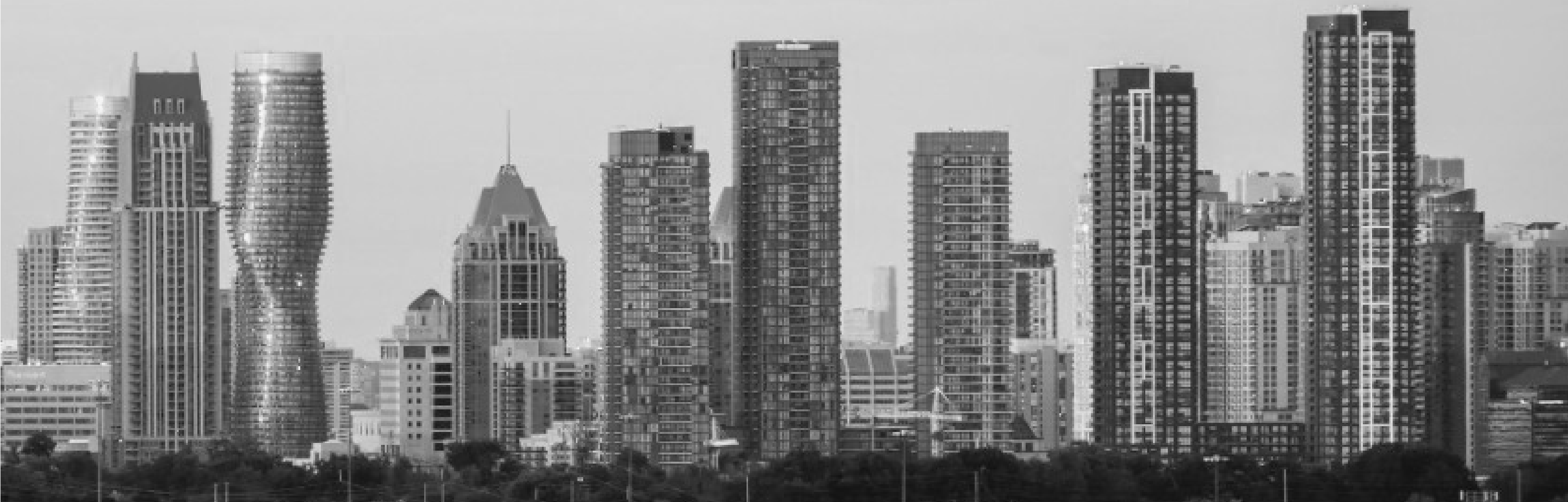
Image of Mississauga's skyline encompassing a diversity of high rise building forms.
