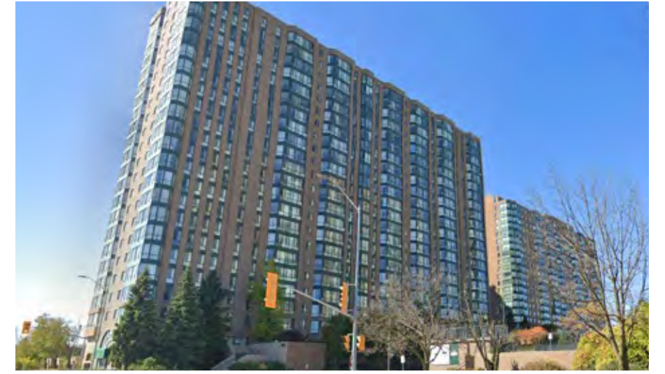
3 View of The Carlyle Condominiums looking west from Hillcrest Avenue
