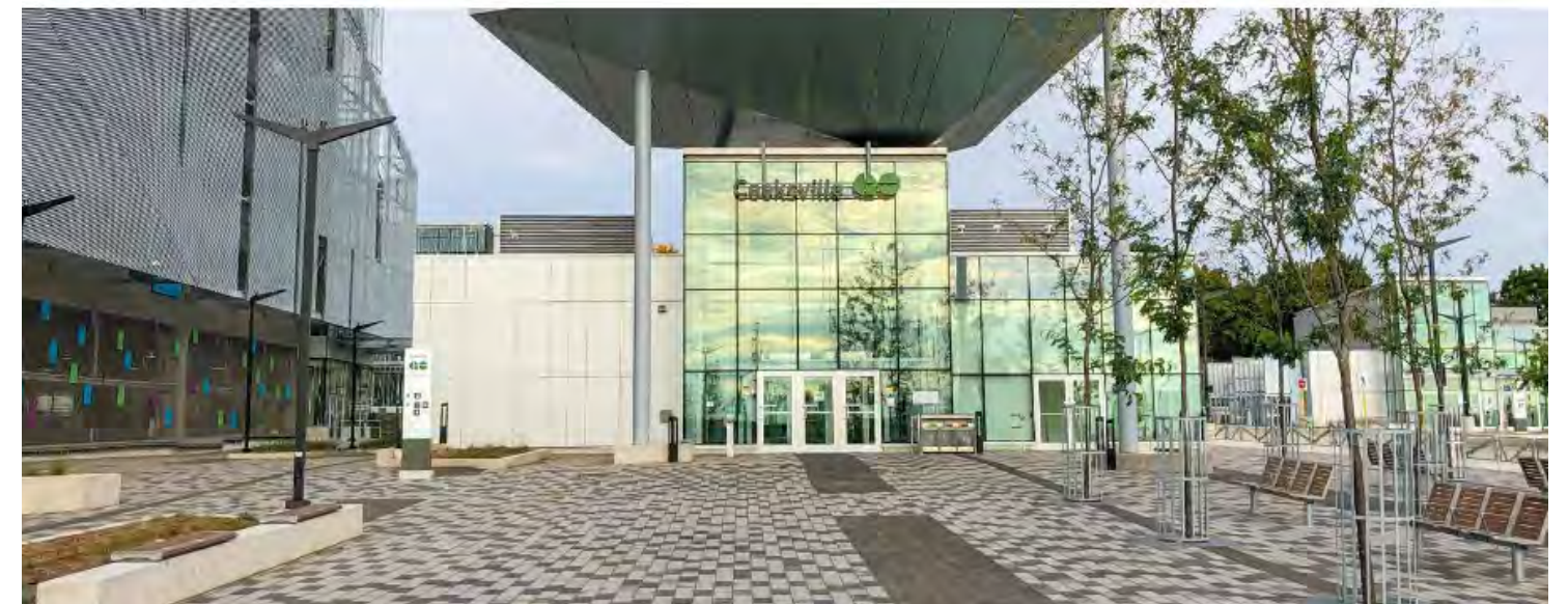
View of Cooksville GO Station
