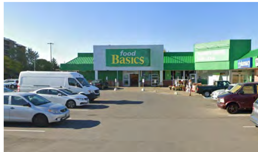
8 Existing Food Basics grocery store facing south west along Hurontario Street
