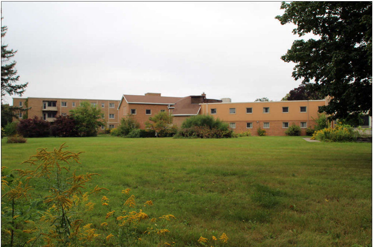
Figure 16 rear of building, south side
