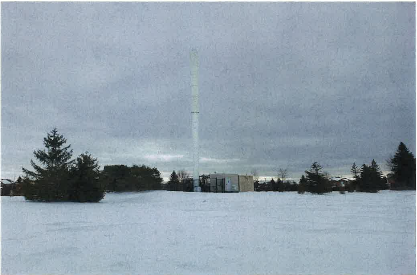
General view of a cell tower and the southeastern boundary of the subject site, facing north
