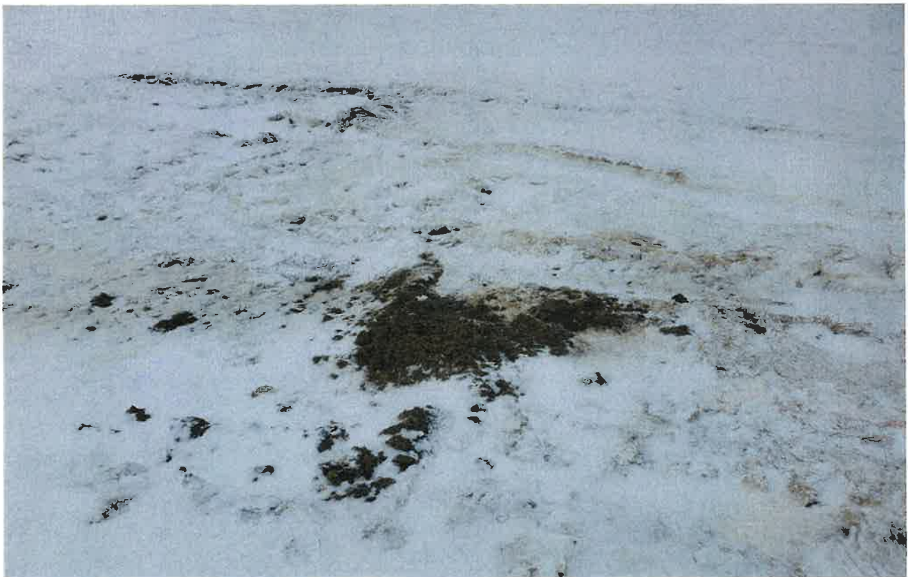
View of boreholes completed by the SEL Geotechnical department on February 24, 2023
