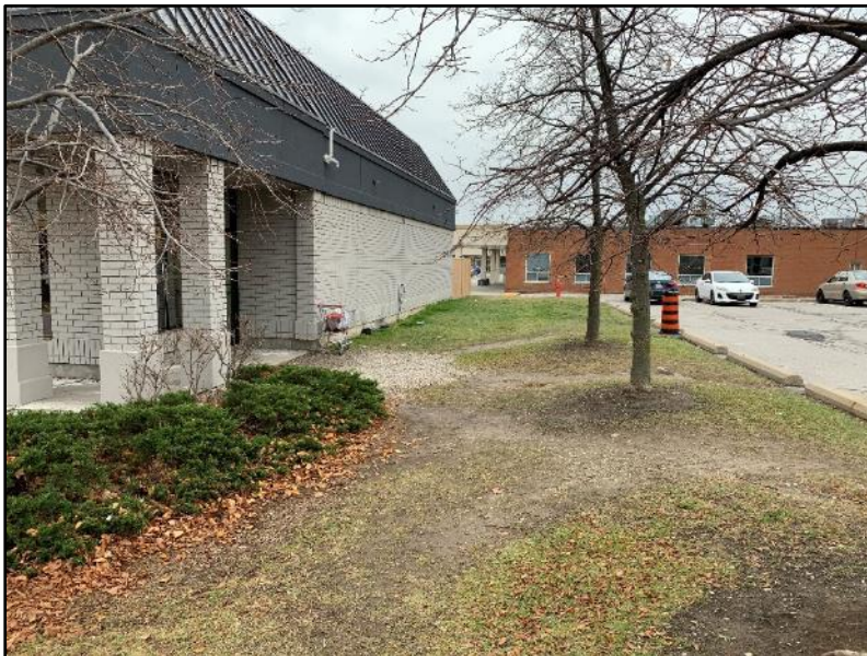
Image 10: Side view of northern commercial building and side landscaped lawn with trees and shrubs.
