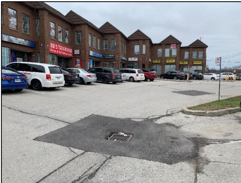
Image 8: A staggered commercial structure on the southeast side of the subject property with a paved asphalt parking lot with a storm water catch basin.
