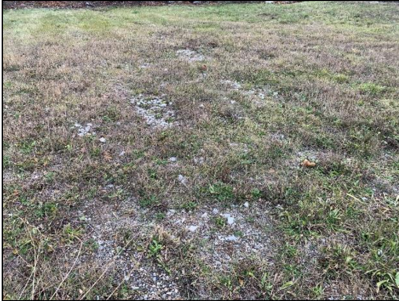
Image 15: Overgrown gravel parking areas on the east side of the subject property, fronting Queen Street South.
