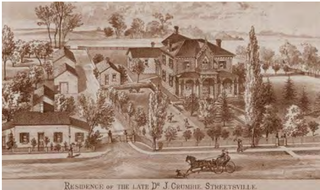
Figure 21: A sketch depicting the main residence of the late Dr. John Crumbie, located on the main thoroughfare of Streetsville (now Queen Street) (Pope, 1877b).
