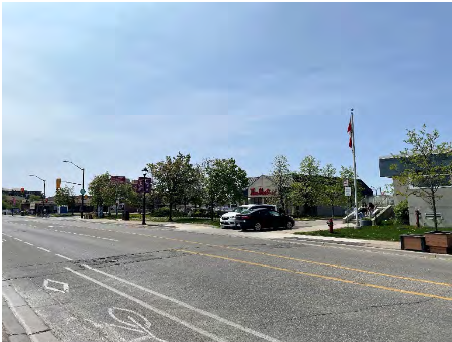
Figure 48: Queen Street South, looking southeast from the northern end of the 1960s commercial plaza. The subject house is visible on the far left (A.S.I., 2023).
