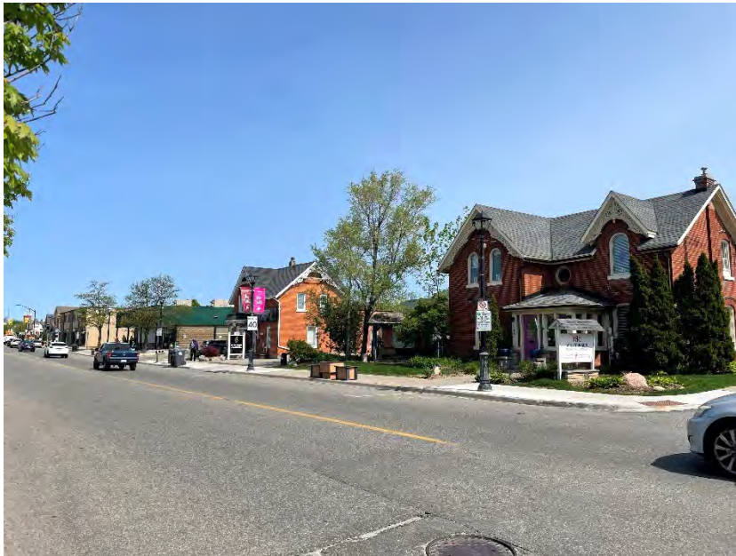
Figure 18: The east side of Queen Street South opposite the project site, looking north from just south of the pub (A.S.I., 2023).
