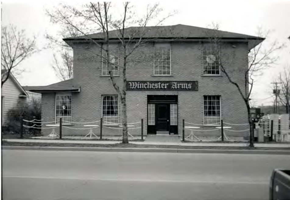
Figure 35: The house at 158 Queen St., 1982 (Mississauga Library Photo Galleries)
