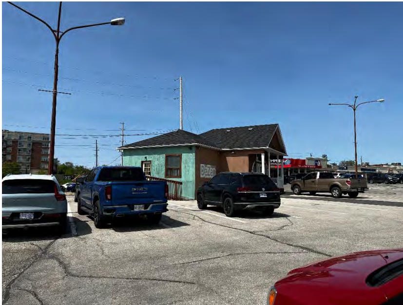
Figure 14: The temporary development office in the site parking lot, looking northeast (A.S.I., 2023).
