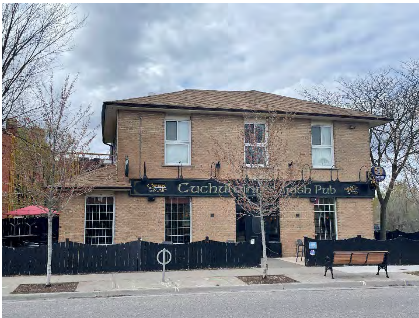
Figure 36: The front (east) elevation of the pub at 158 Queen Street South (A.S.I., 2023).
