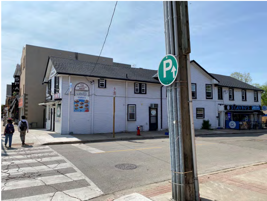
Figure 52: Intersection of Queen and Main/Pearl Streets, looking south with 210 Queen St s. in the foreground (A.S.I., 2023).
