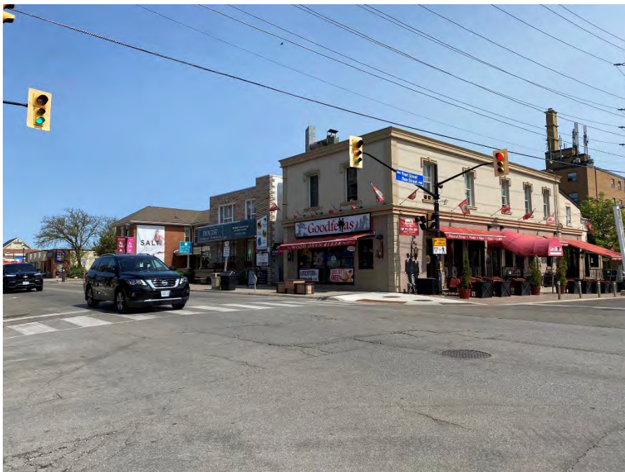
Figure 53: Intersection of Queen and Main/Pearl Streets, looking north towards the east side of the street (A.S.I., 2023).
