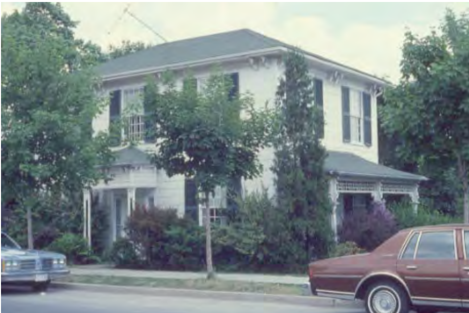
Figure 34: The house at 158 Queen St., 1978 (Mississauga Library Photo Galleries)
