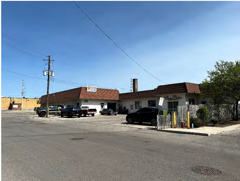
Figure 12: The commercial building at the southwest corner of the site, looking north (A.S.I., 2023).
