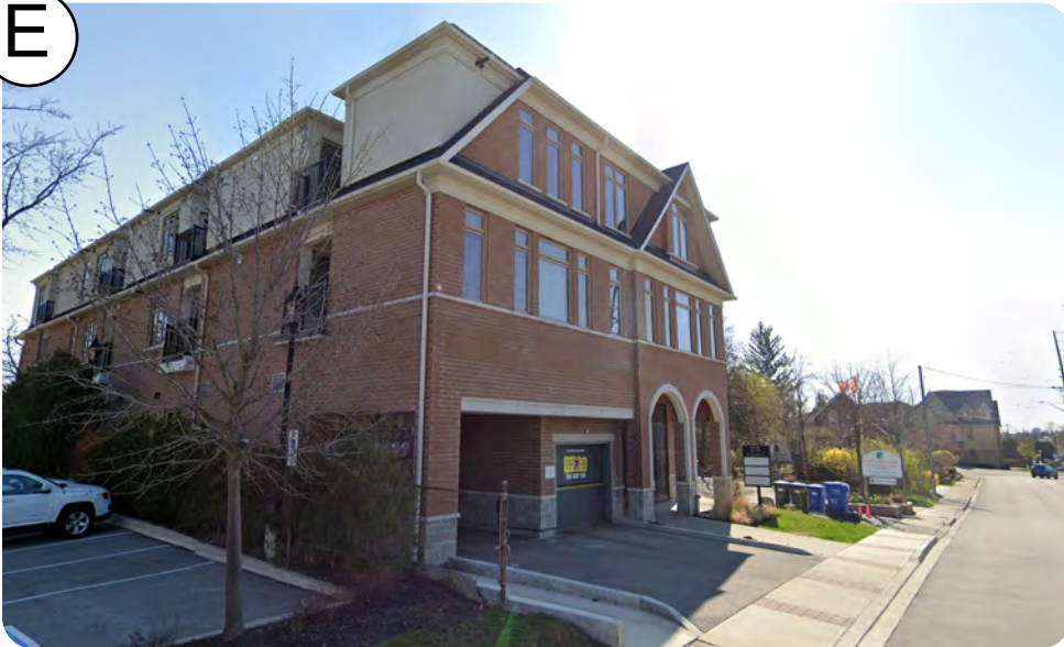
215 Broadway Street Source: UrbanTO
