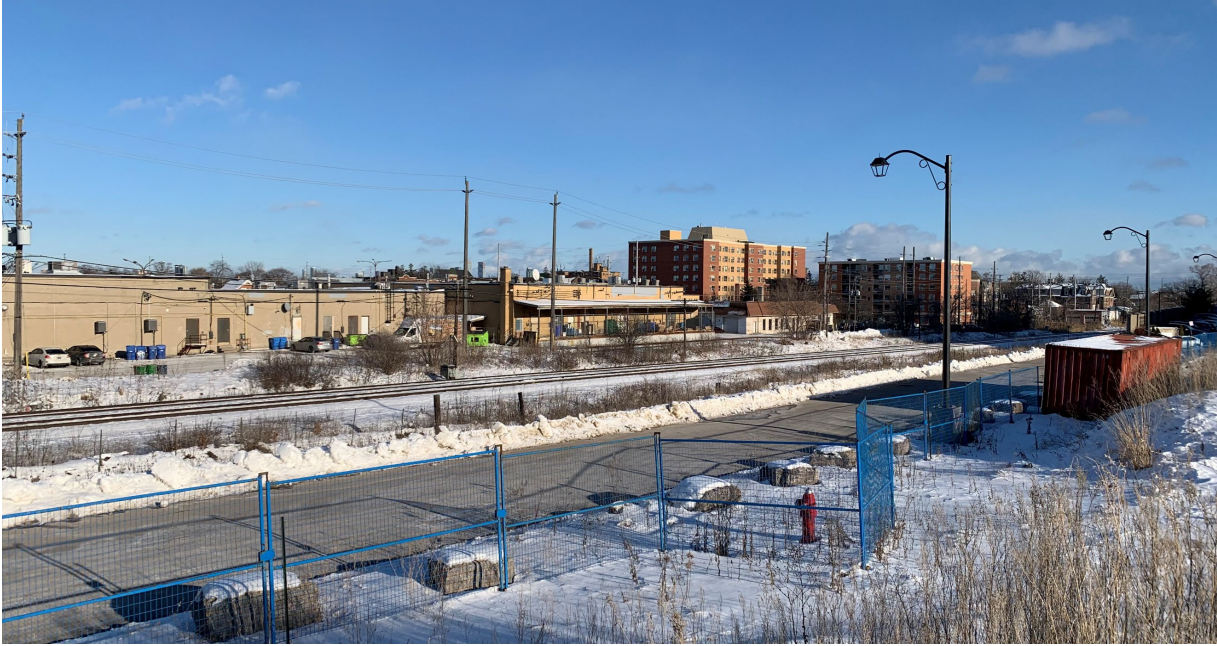
Photo 5 View of Rutledge Road and railway east adjacent to Site, facing east
